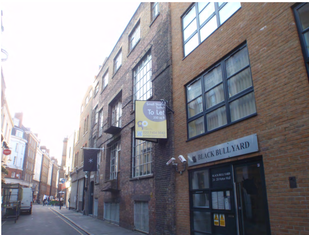
View of front elevation and entrance to 24 – 28 Hatton Wall, Black Bull Yard.
