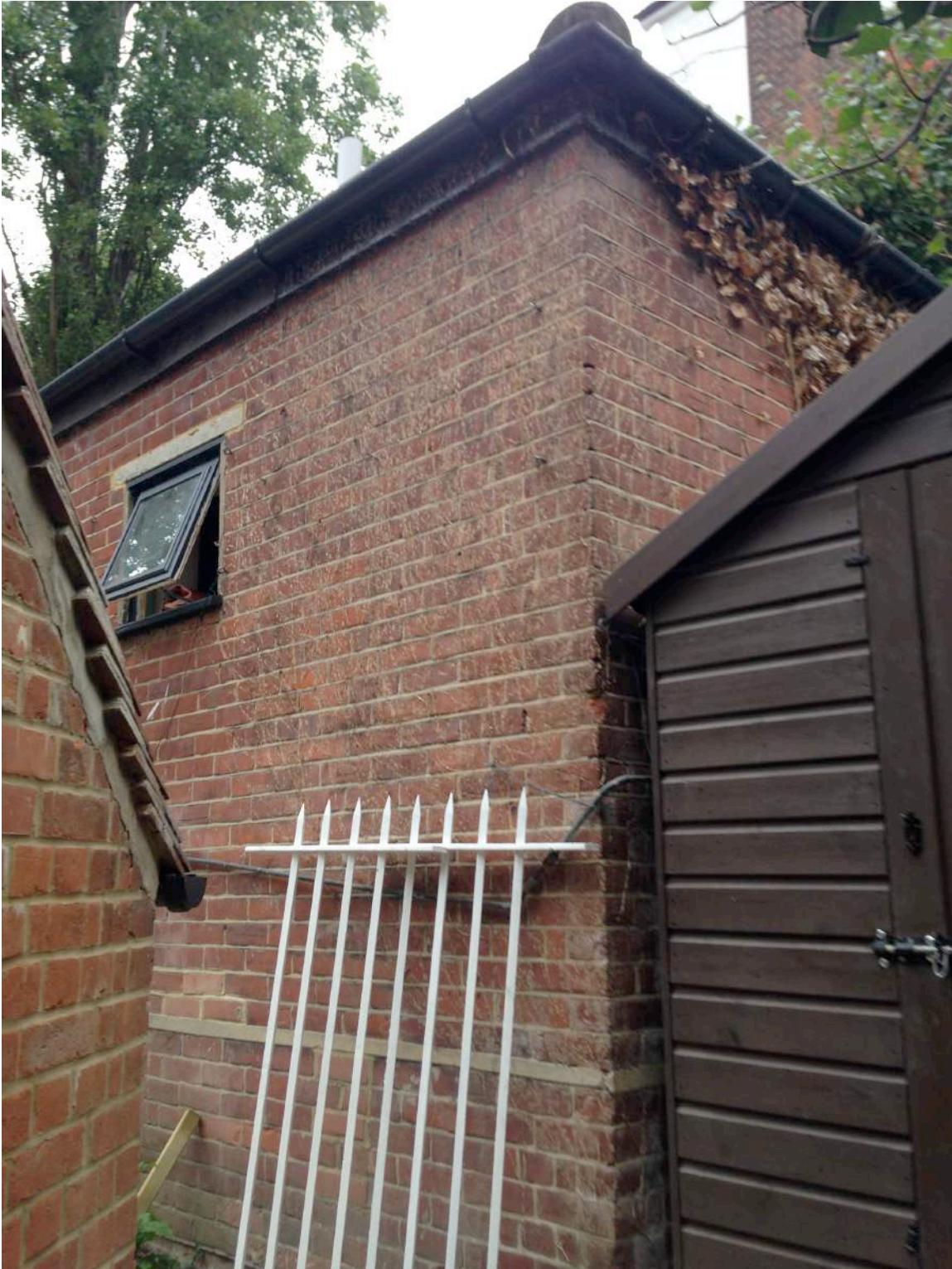
Lower Wellside, view of the rear elevation from Wellside
