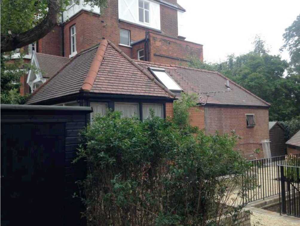
Lower Wellside Side Elevation from Wellside
