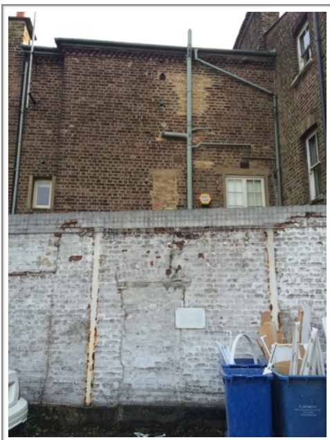
Rear elevation of the existing house and the rear wall.
