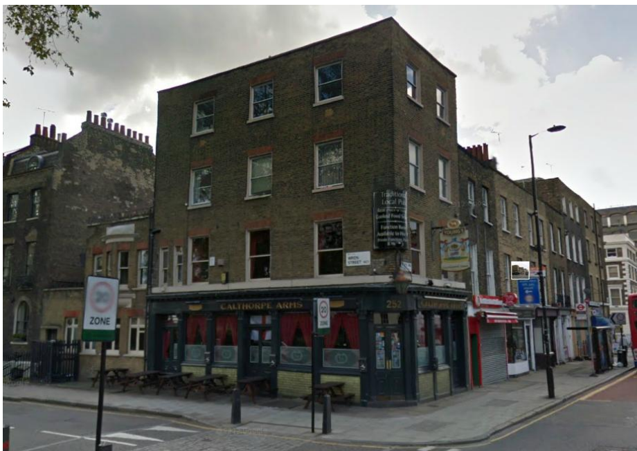
Fig.1 View of the Calthorpe Arms from the north corner of Wren Street
