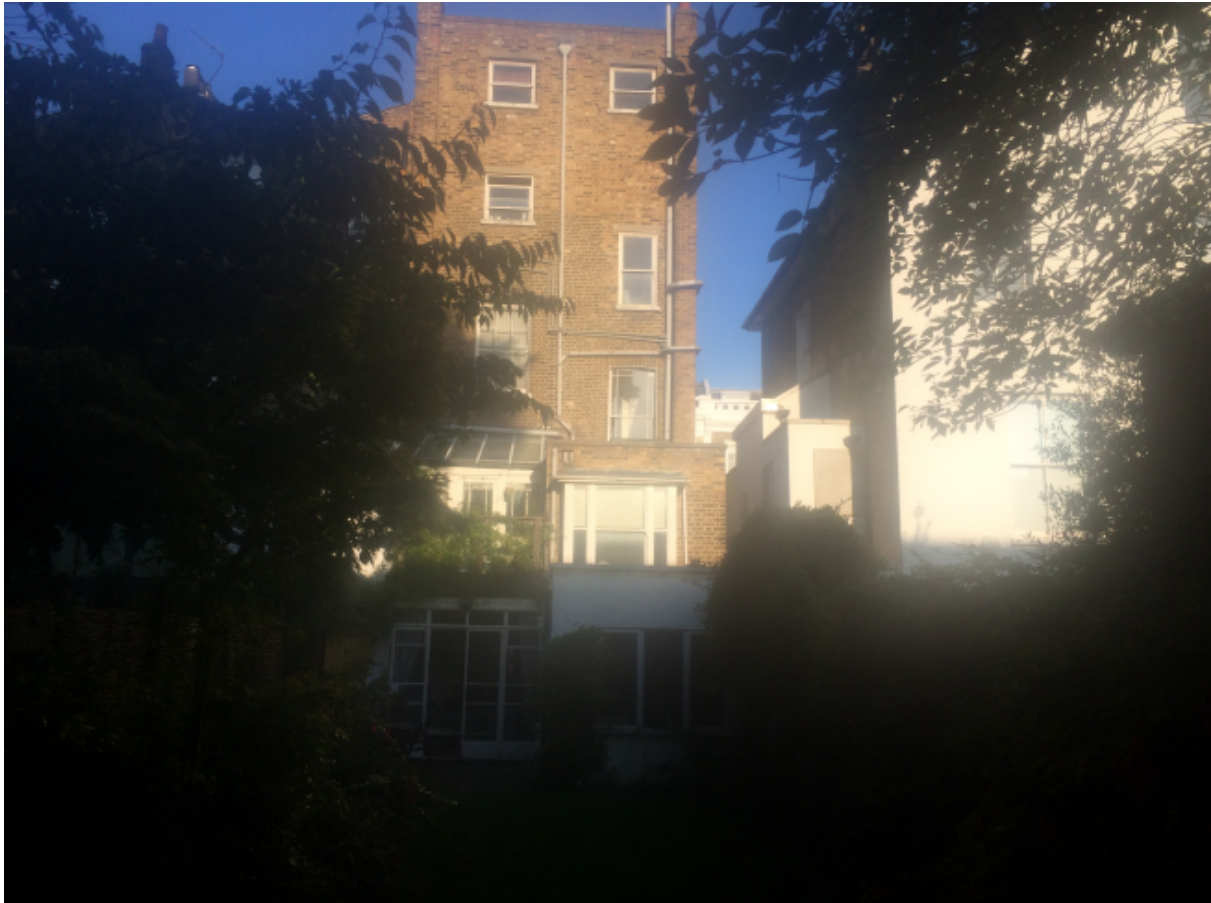
3. Rear elevation of building
