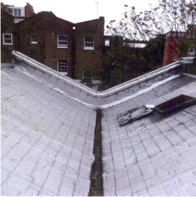
fig19. Roof with 'flashband' covering
