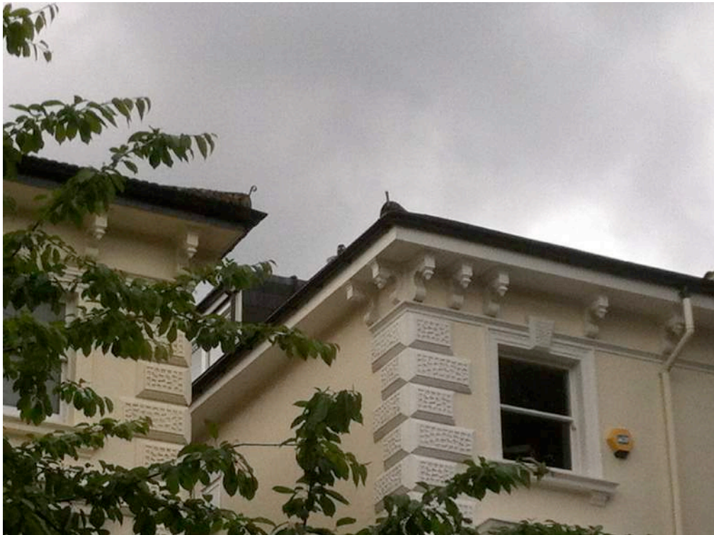
8 Belsize Square Side Dormer View
