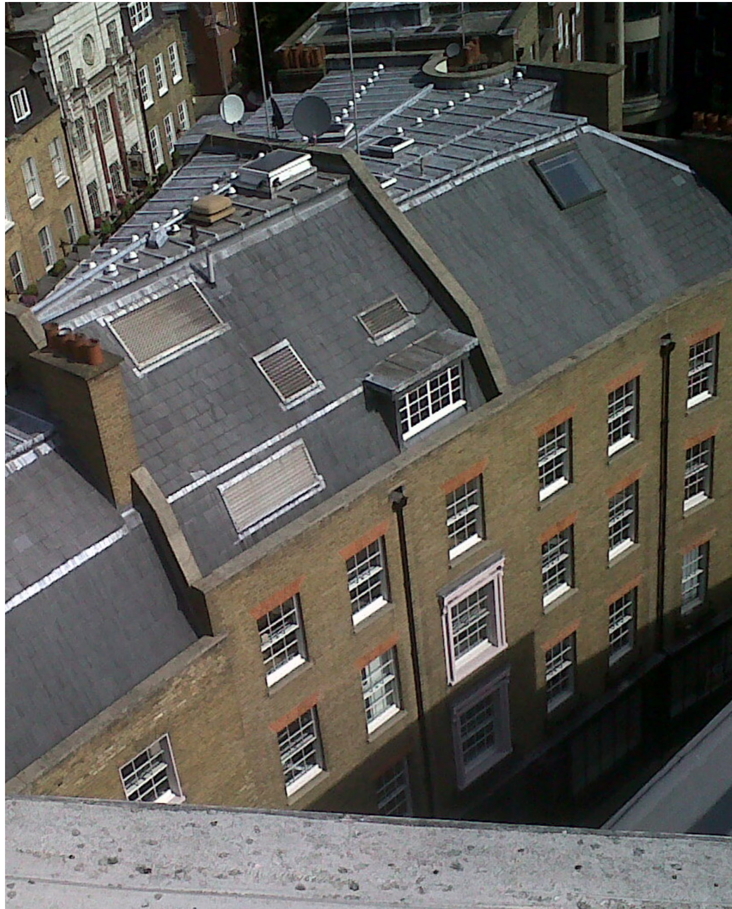
01. 65 - 75 Monmouth Street - Photograph of the existing roof
