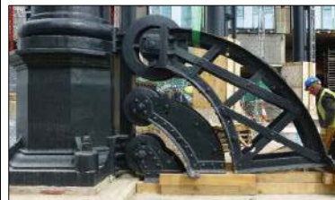
Image illustrates site mockup of roller arrangement, 01.04.2015
