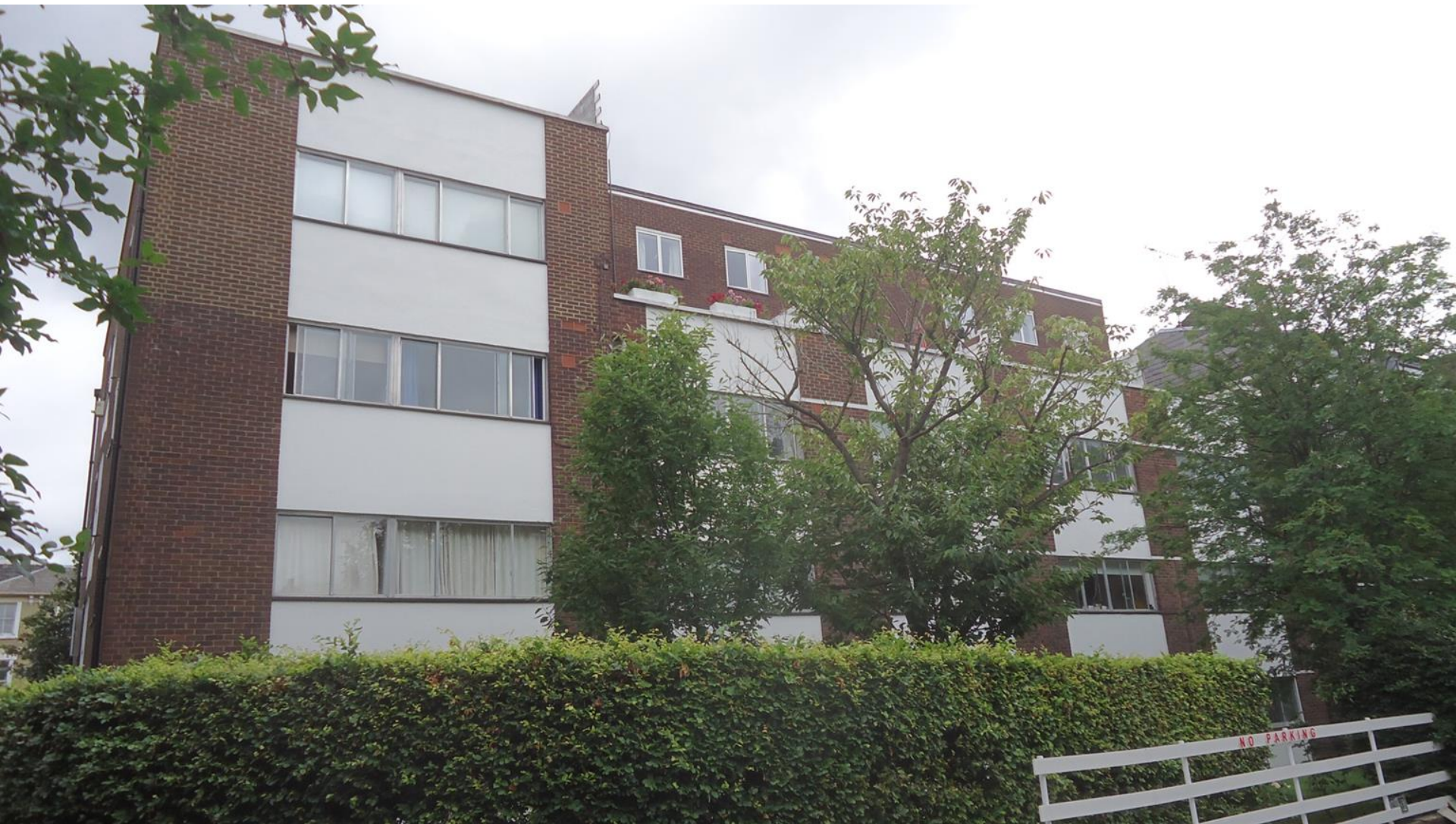
SW FAÇADE REAR
