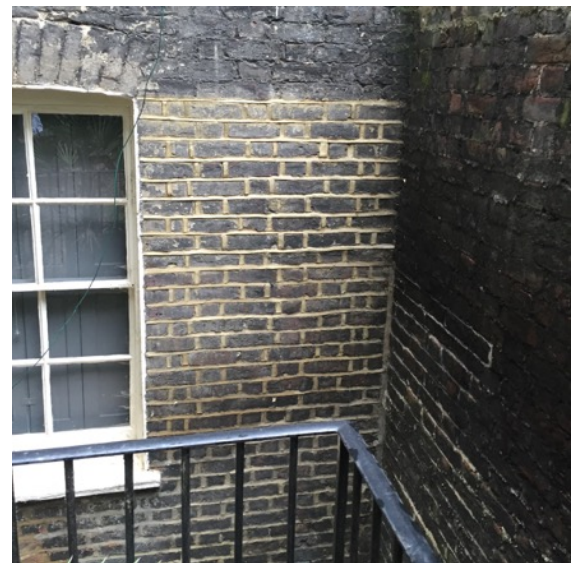
Rear Wall Previous Repointing Works
