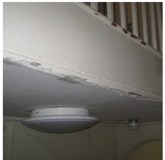
Ceiling Beneath Third Floor Landing
