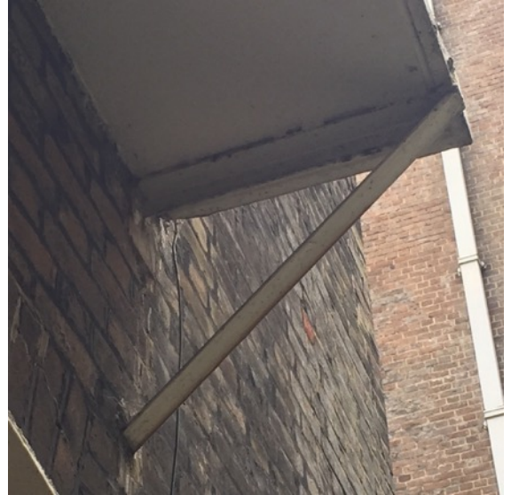
Rear Balcony Brackets
