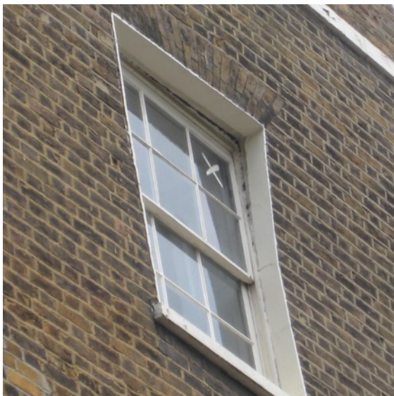
Close Up View of Front Facade
