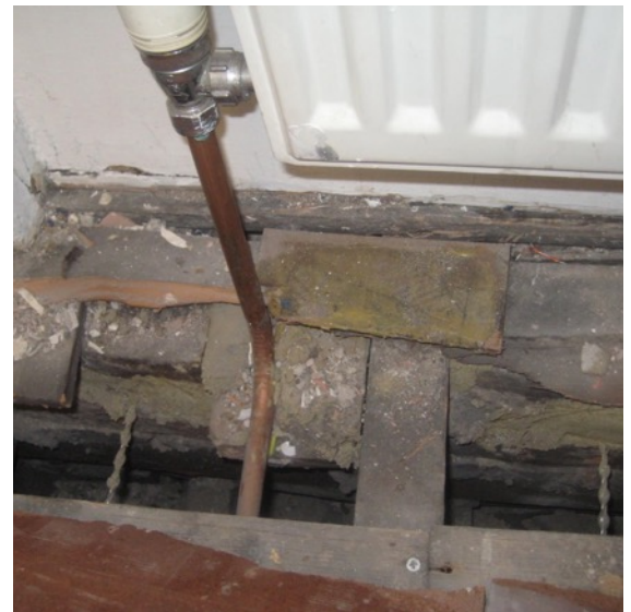
Third Floor Steel Helical Ties in Wall
