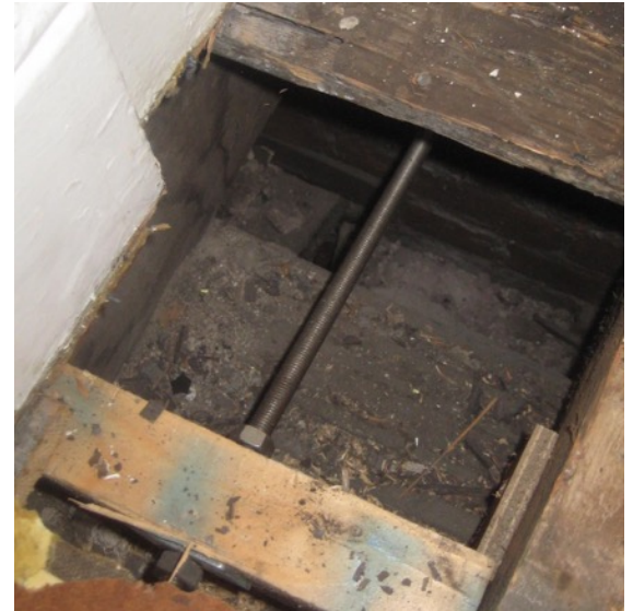
Second Floor Wall Ties
