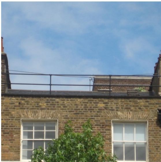
View of Chimney Stacks and Tie
