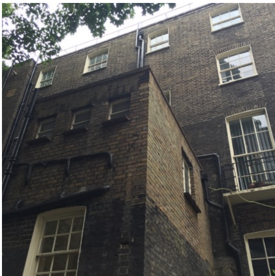
View of Rear Extension
