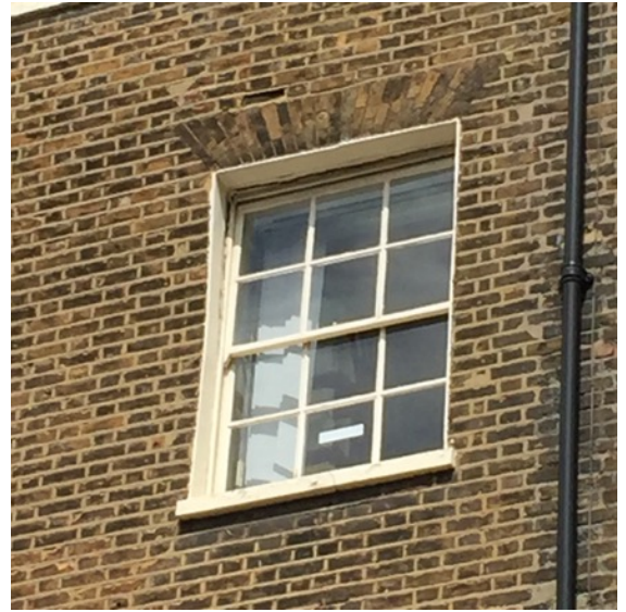
Close Up View of Front Facade
