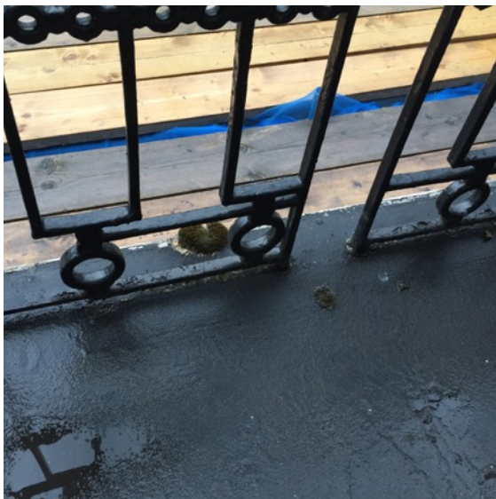
Close Up View of First Floor Balcony
