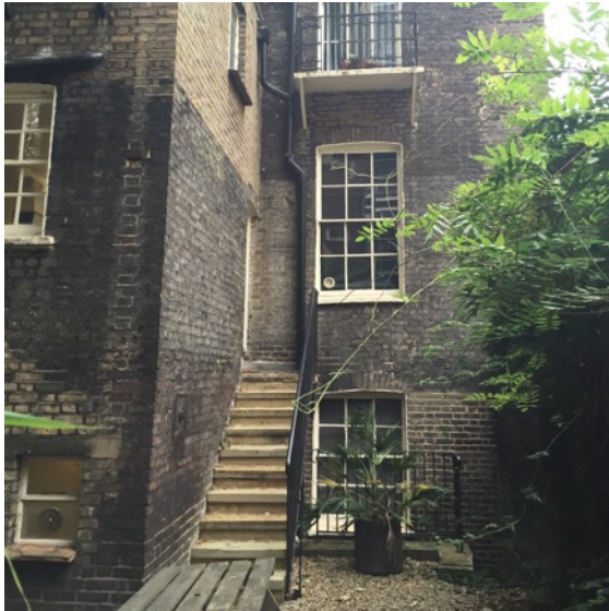
Rear View of the Property
