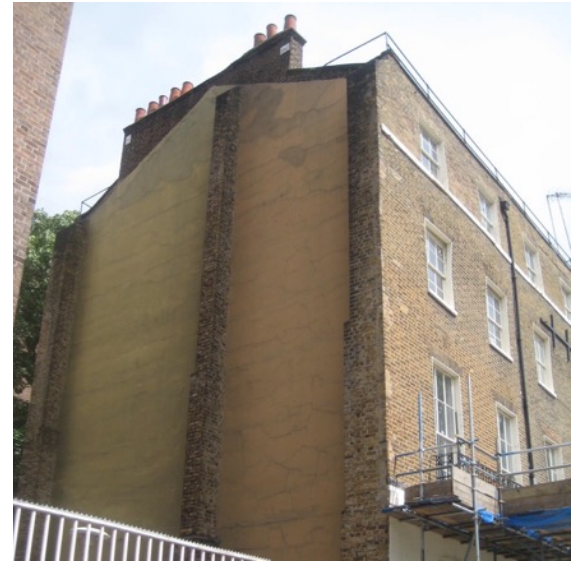
View of Flank Wall
