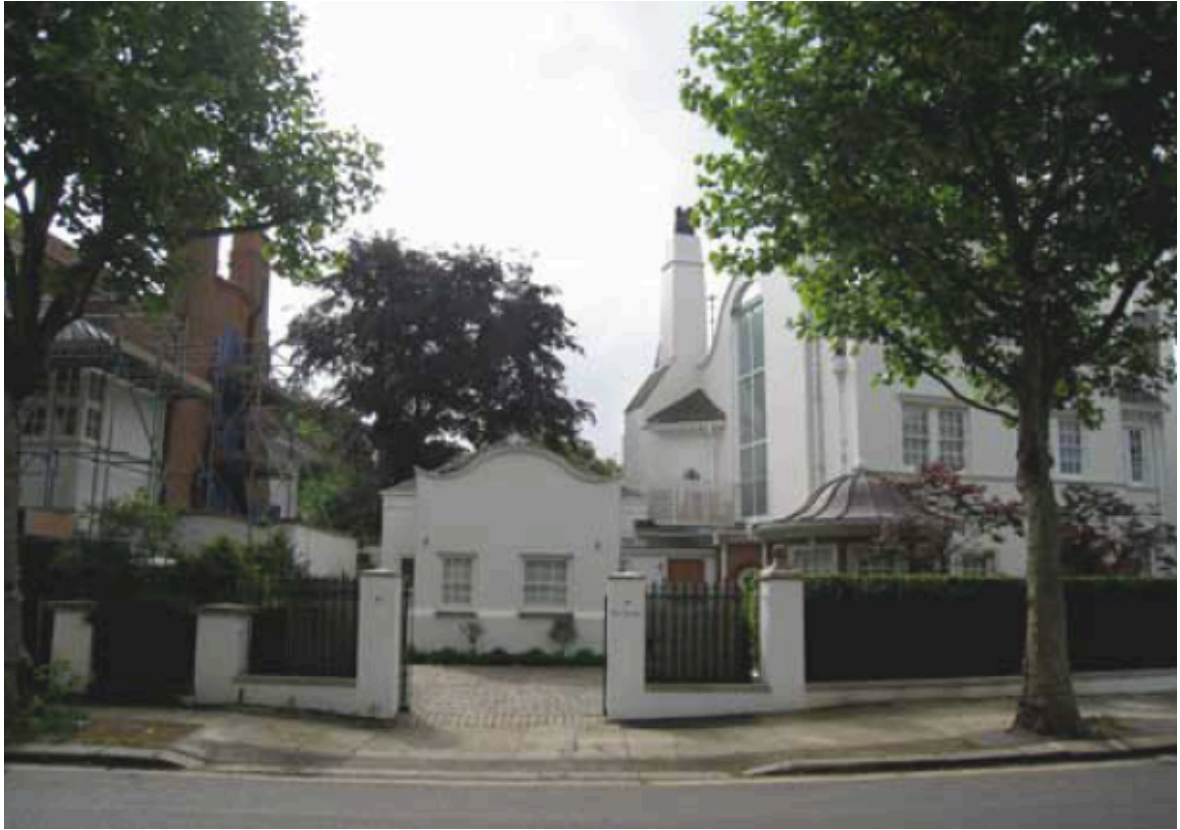
Photograph 1: Street View of 4a Wadham Gardens and driveway entrance
