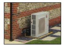
heat pumps are between 200% - 400%. Heat pumps can operate at outside temperatures down to -15 degC, although there is a drop in COP.
