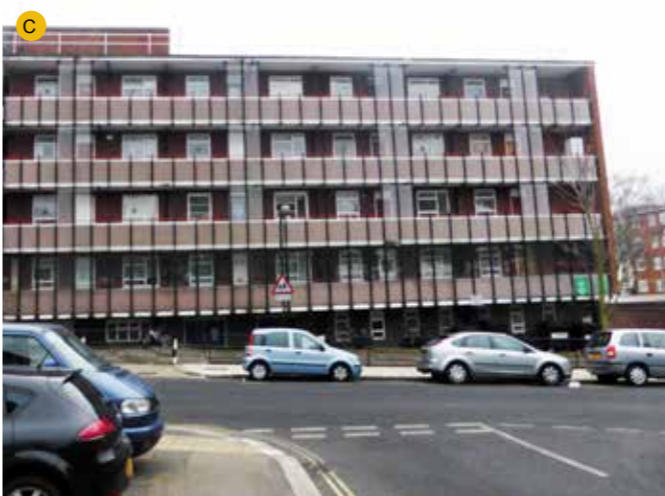
4&5 storey Holmesdale House opposite the development site (part of the Kilburn Vale housing estate)
