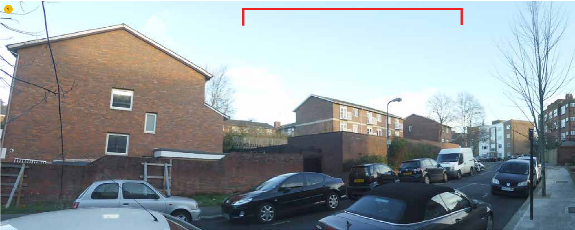
The view up West End Lane towards the site along the south elevation of the garages
