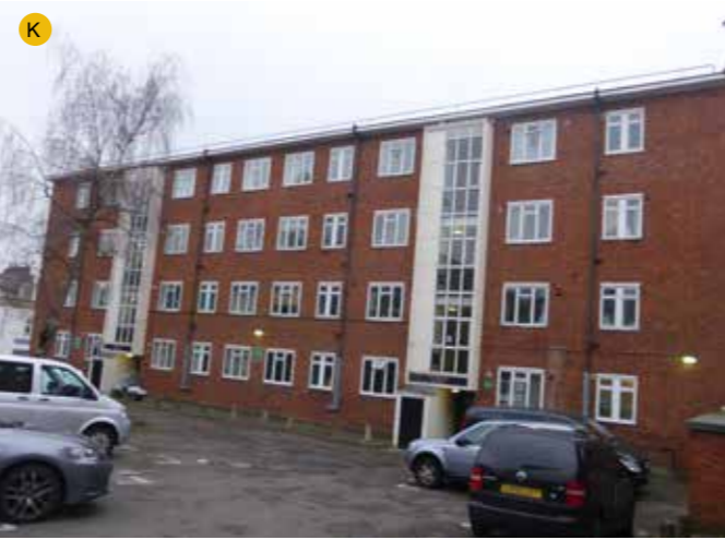
Farnedale House, 4 storey block of flats
