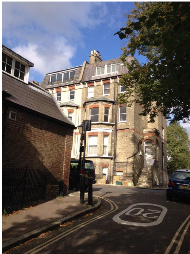
Photo 2: Front elevation looking north from Cannon Lane
