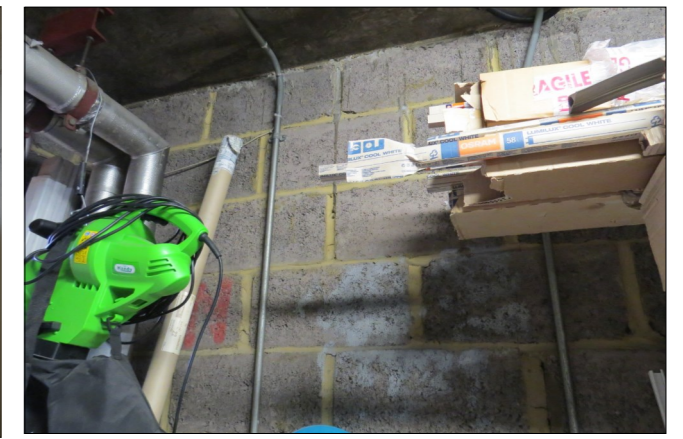
10—Location of proposed penetration in rear room
