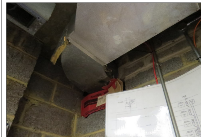
7—Existing plant penetrating rear wall of first room
