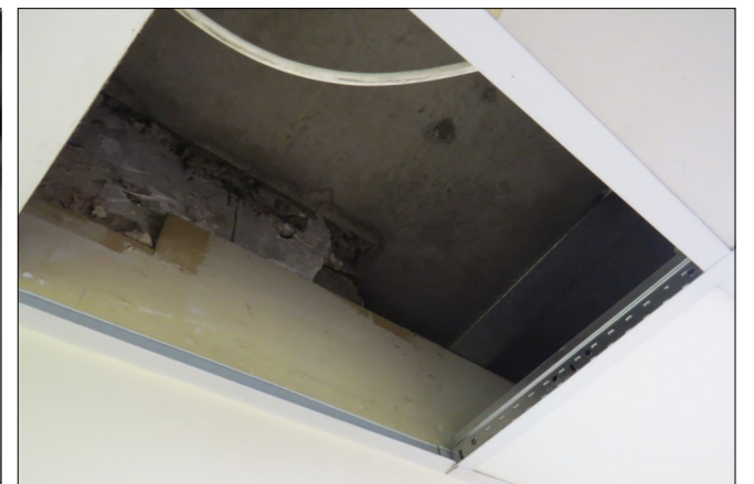
14—Above suspended ceiling in image 13
