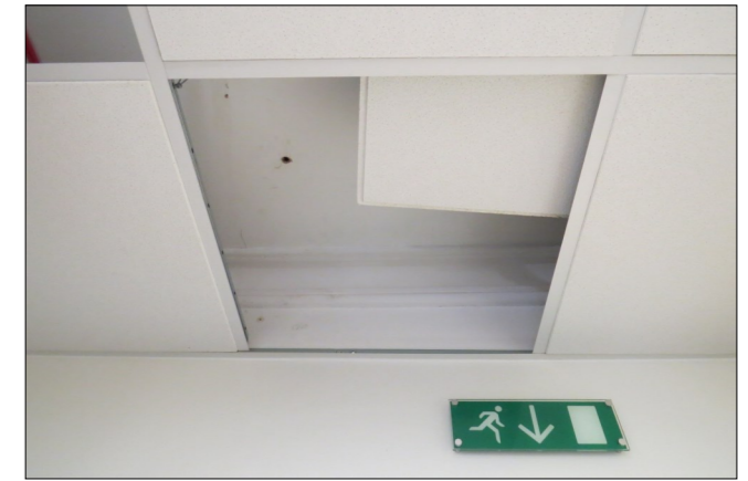
2—Cornice concealed by suspended ceiling
