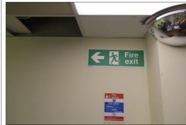
13—Location of proposed penetration, wall not original
