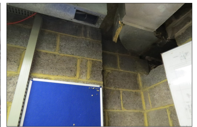
12—Location of proposed penetration in first room
