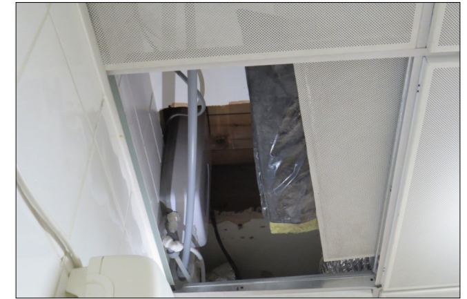
4— Floorboards and plant above suspended ceiling
