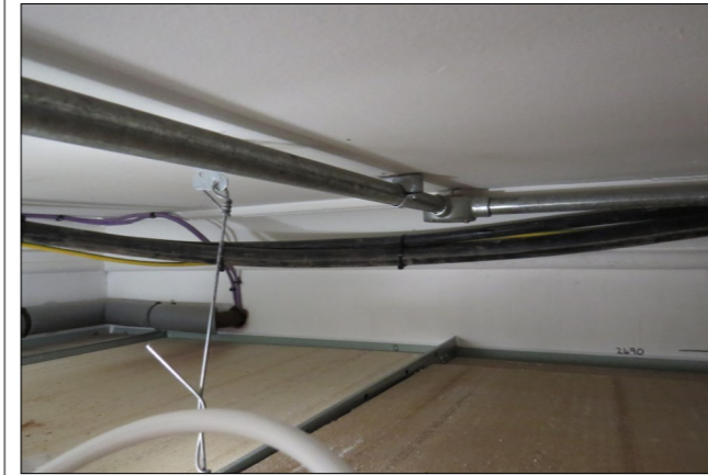
3—Cornice and existing penetration of wall
