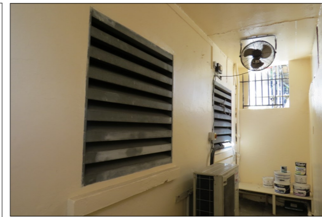
9—Louvre in external corridor of rear plant room
