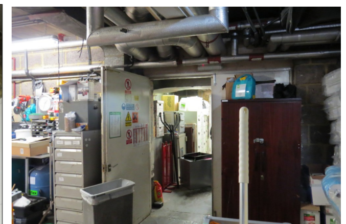
8—General character of the basement plant rooms
