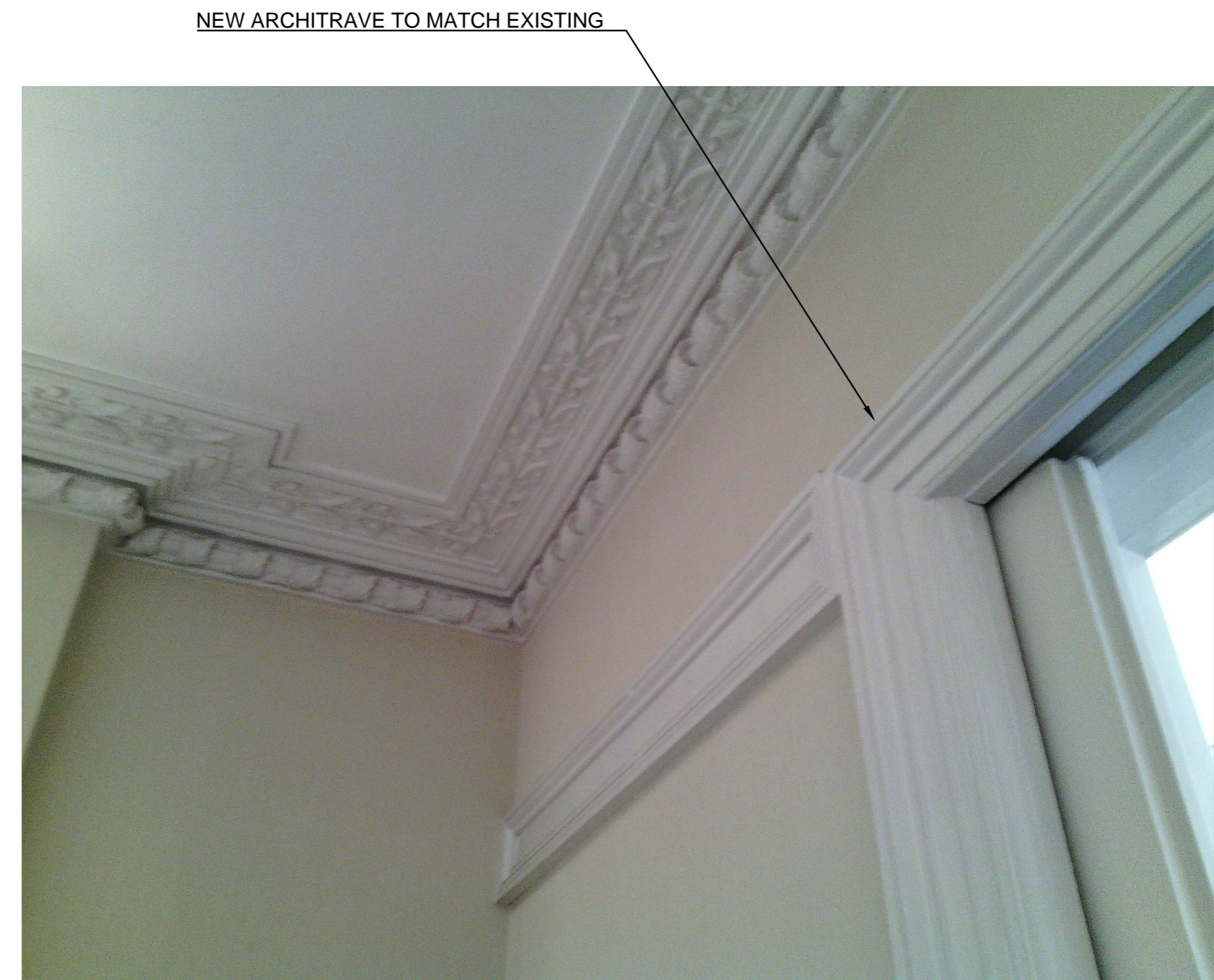
3 EXISTING LISTED BUILDING ARCHITRAVE NTS
