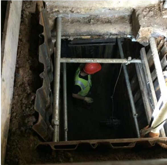
Figure 3 Excavation of Pin
