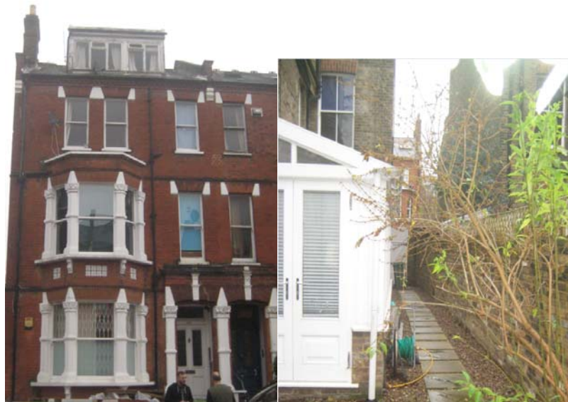
Figure 16: Front and Rear of 106 Savernake Road
