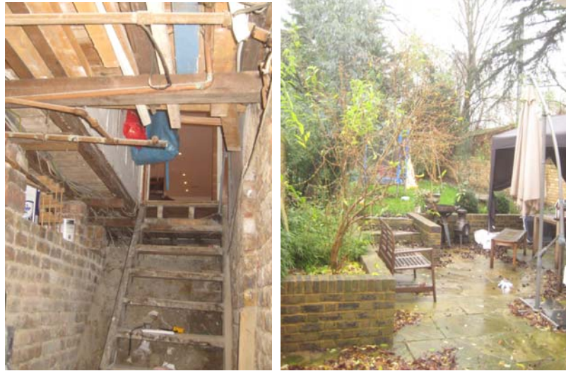
Figure 17: Cellar and back side garden of 106 Savernake Road
