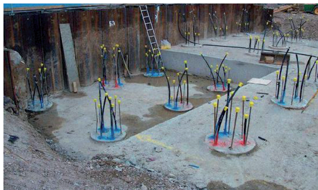
Energy piles within foundations of construction. Source: Geothermal International Italia
