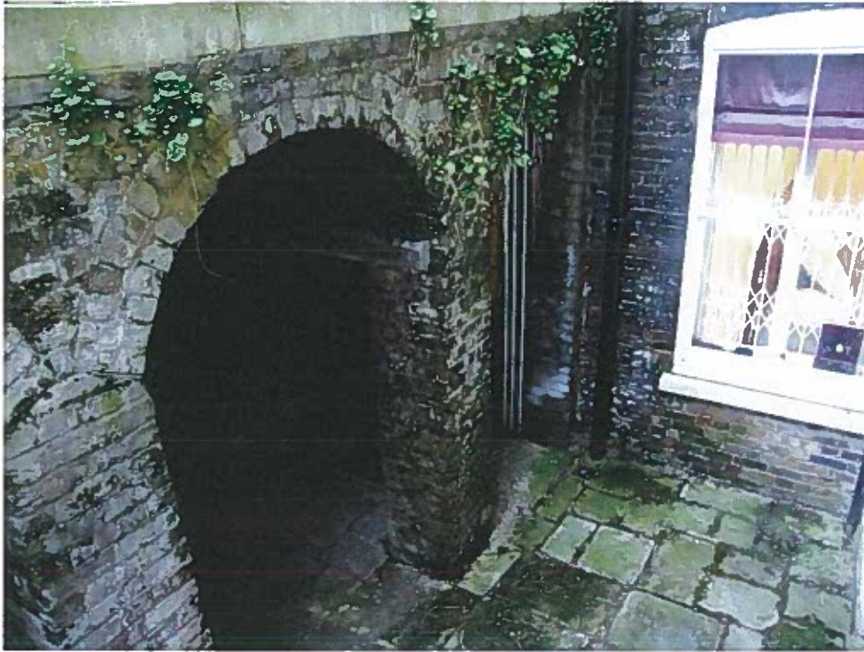
Photo 1 Right hand wing of the external basement
