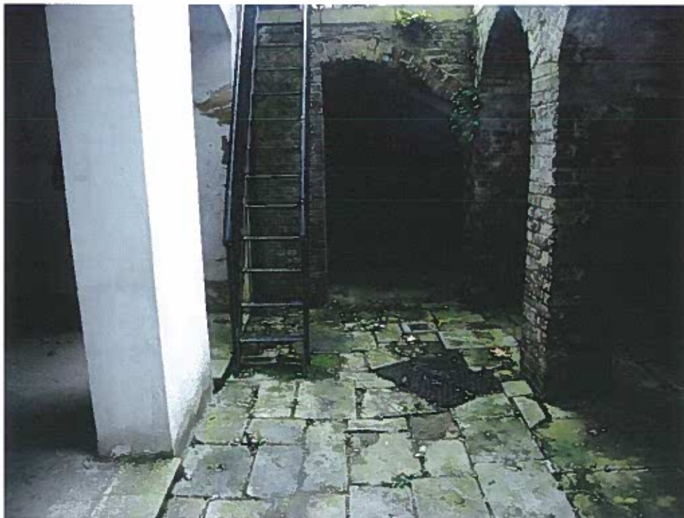
Photo 4 Rear vault of the external basement
