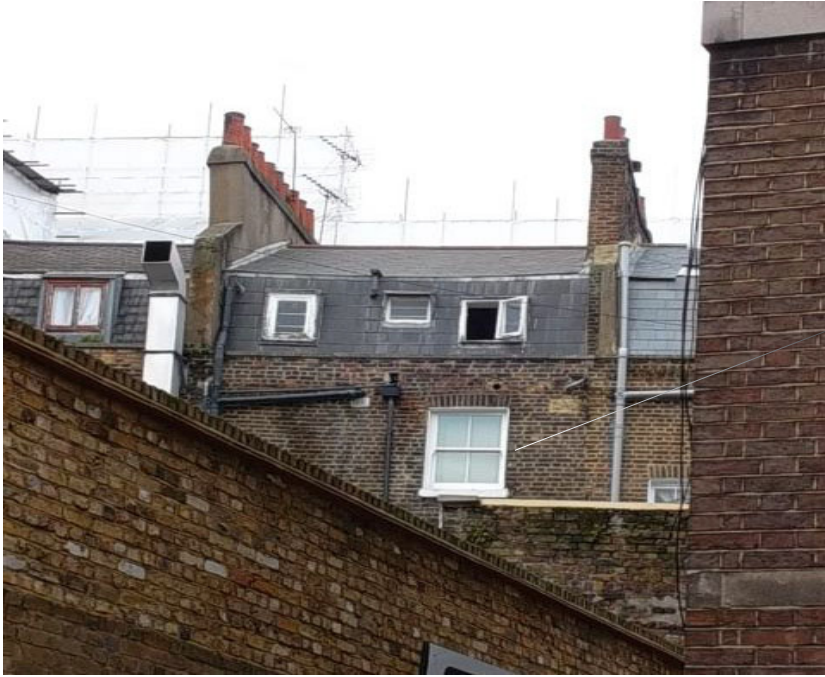
rear view showing existing sash window in floor below
