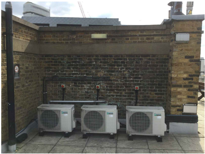
Photograph of existing area
