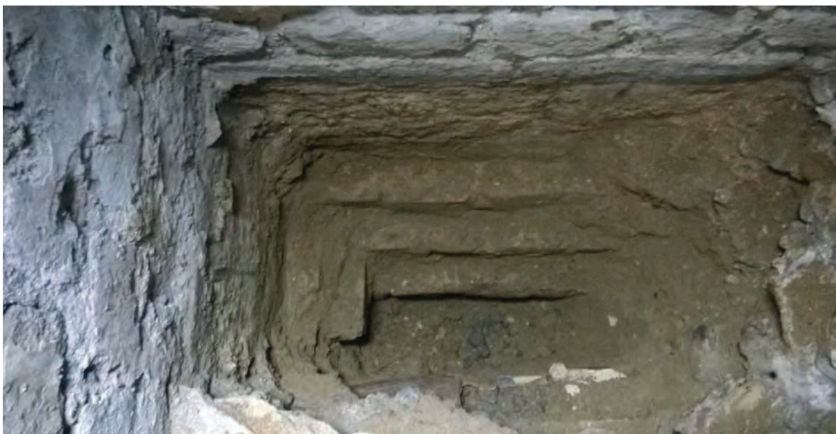
View of Trial Pit No 8
