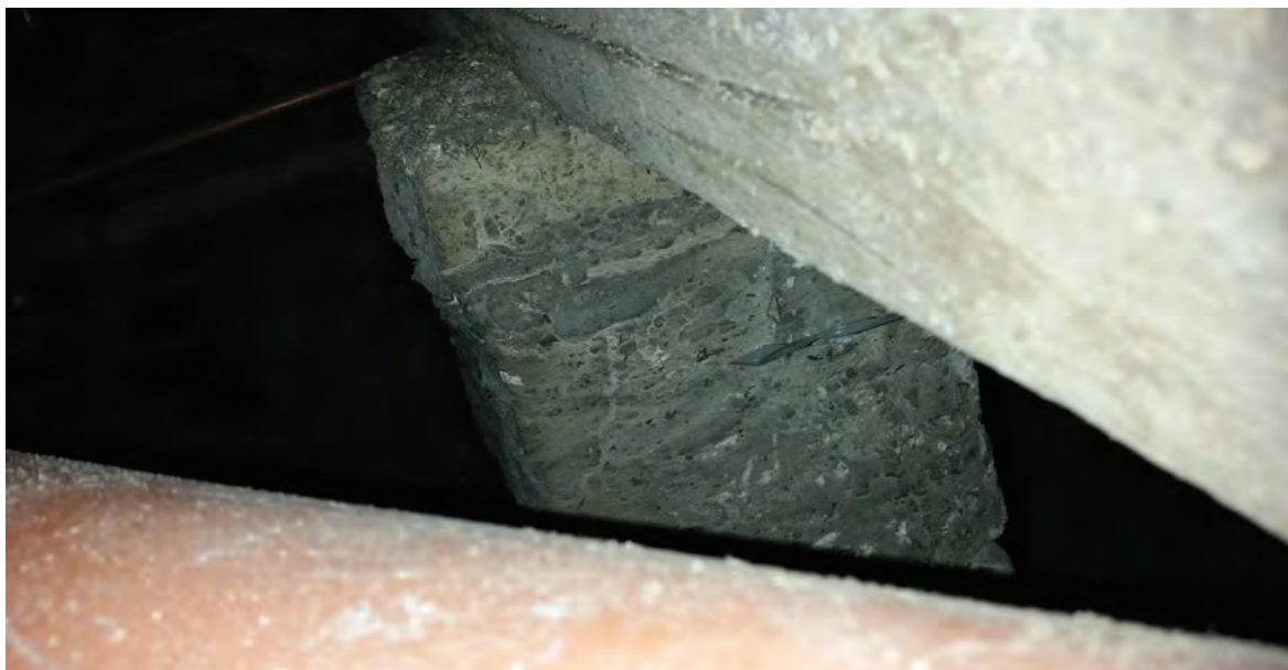
View of brick pylon supporting wooden cross beams
