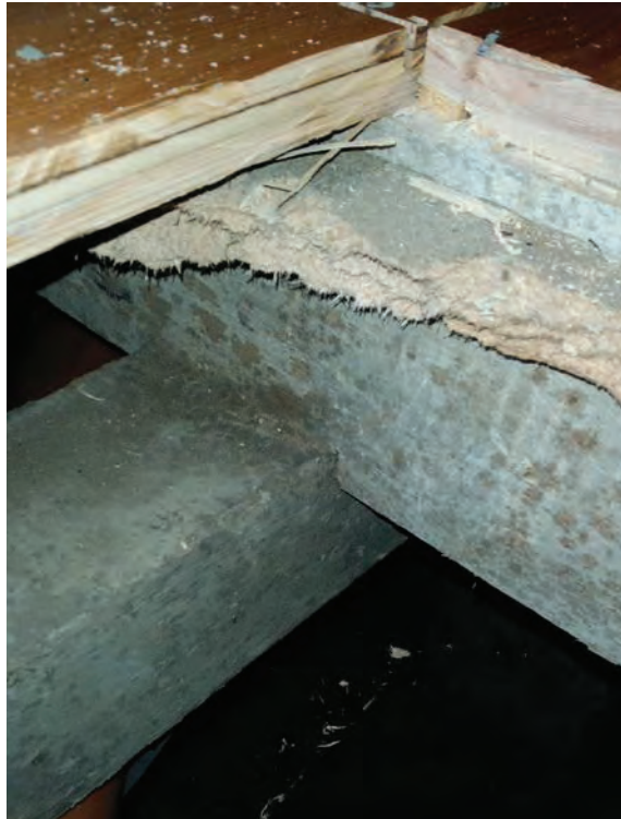
View of concrete beams being supported by wooden cross beams, and the formation of the wooden floor
