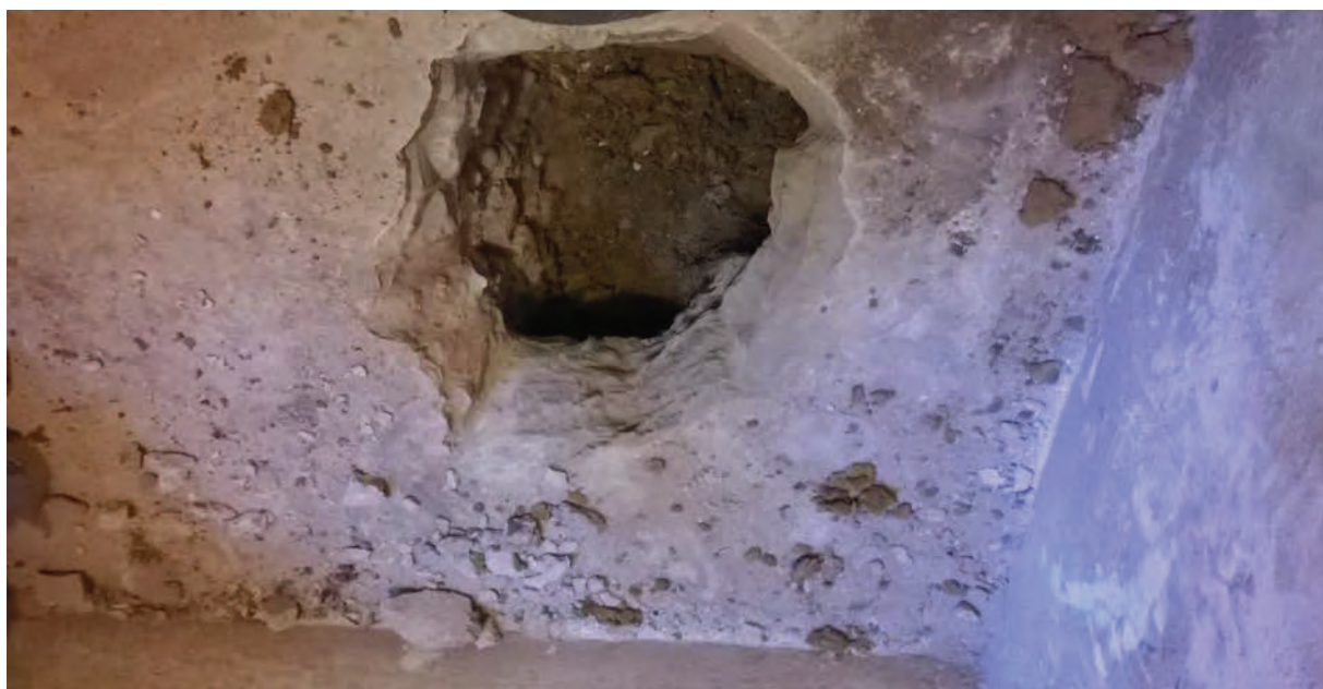
View of Trial Pit No 10
