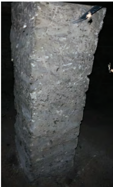
View of brick pylon supporting suspended wooden floor
