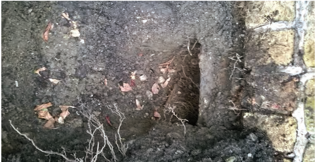
View of Trial Pit No 1
