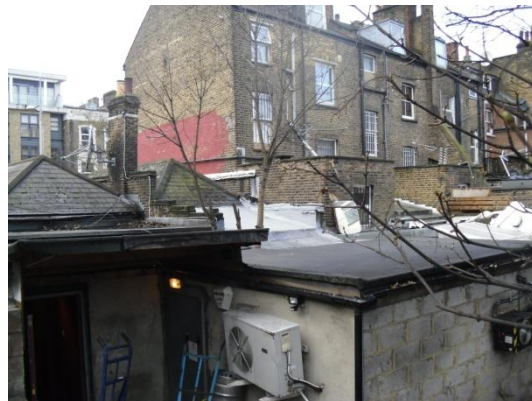
mixture of pitched and flat roofs at rear
