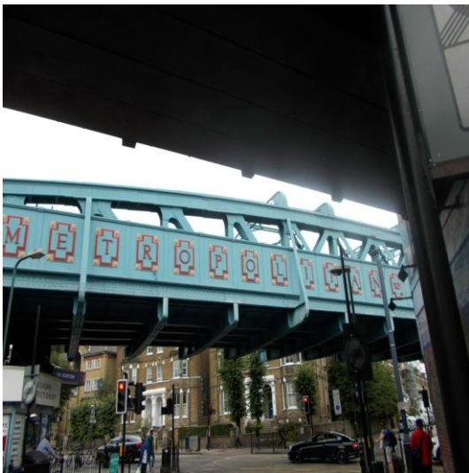
metropolitan railway bridge
