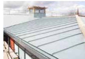
Example of zinc roofing
