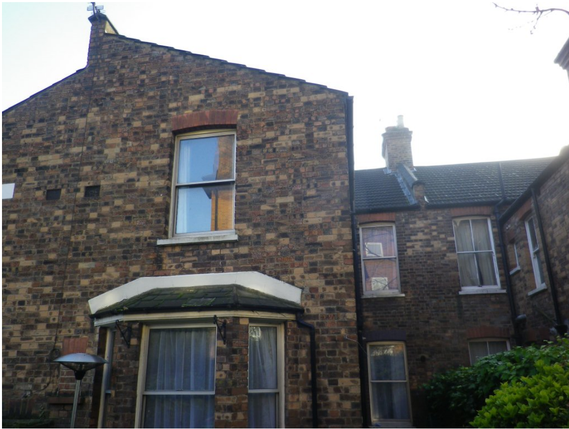
Photograph One: Rear Elevation
