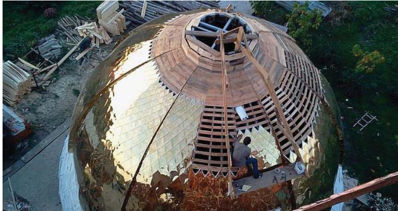
Figure 2-4 Example- use of PVD TiN stainless steel sheets as roof shingles for church domes
