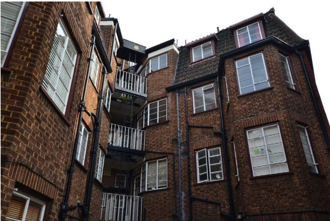
Image 2 – View of rear elevation
