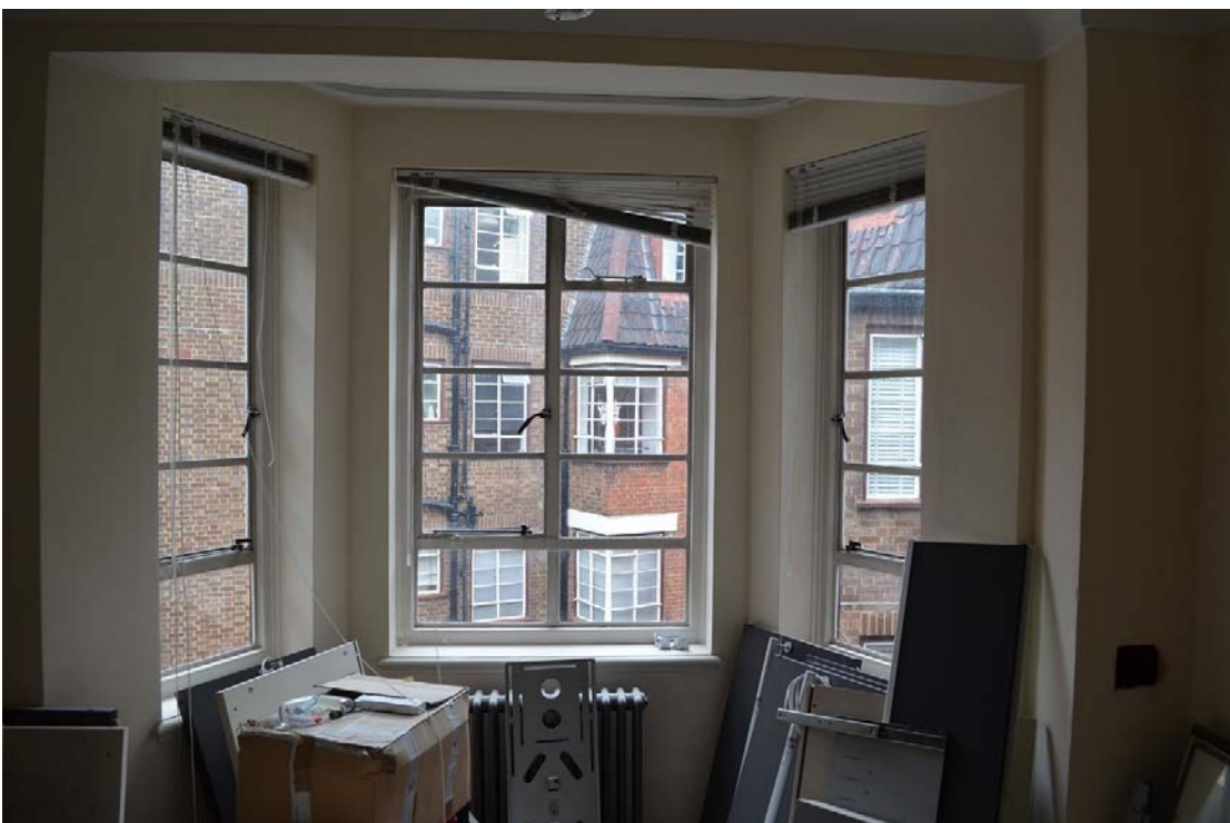
Image 6 – Typical existing window
