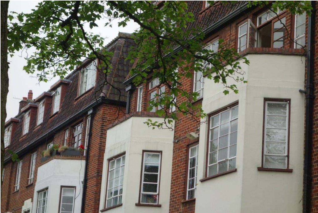
Image 3 – View of front elevation
