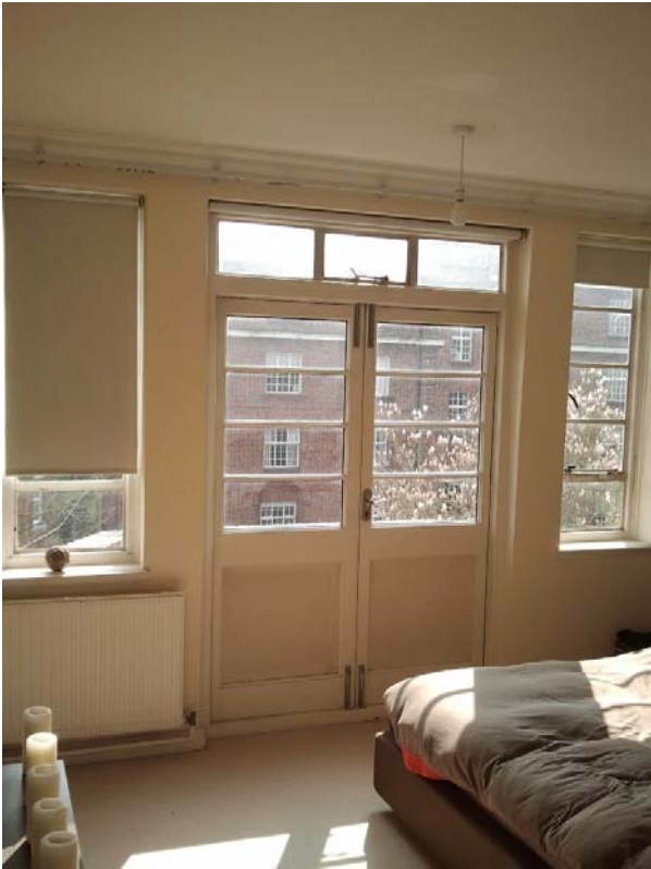
Image 7 – Typical existing door (Not original timber)
