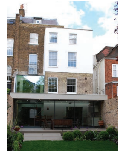
Hamilton Terrace, NW6 - Extension & modernisation of grade II listed terrace house.
