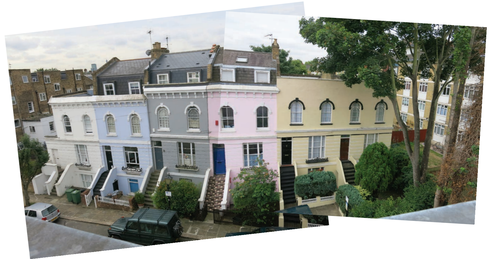
View from second floor of no.8, showing front Facade of South terrace at Baptist Gardens
