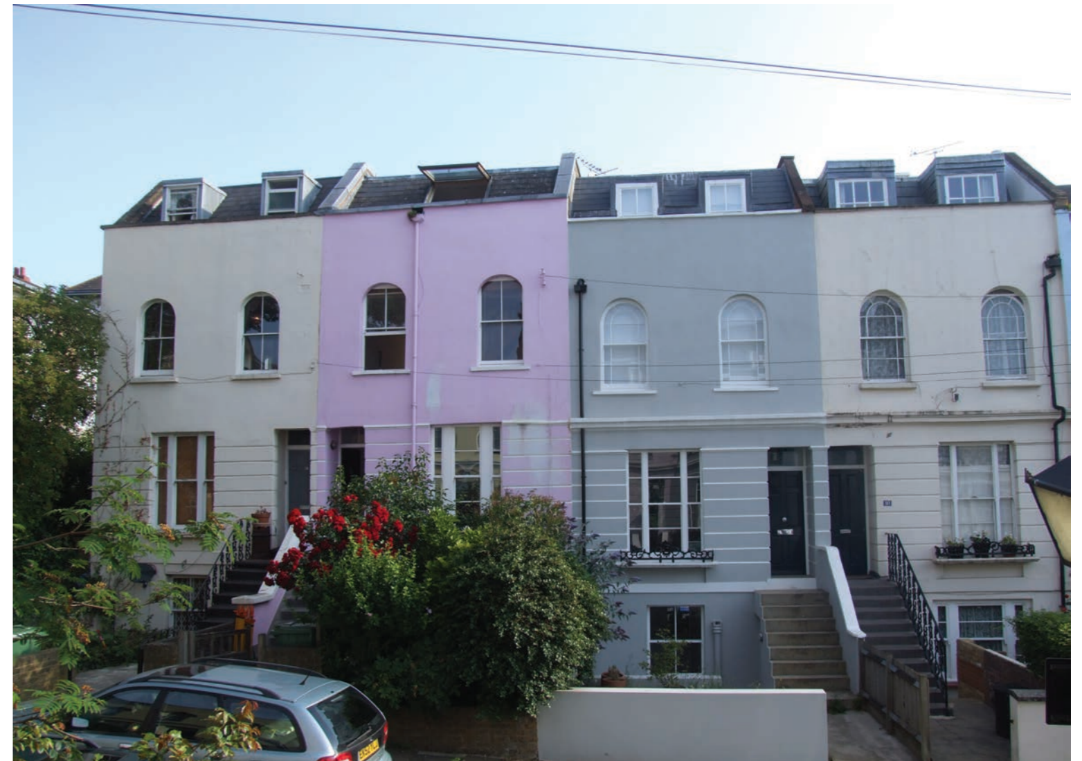
View showing front Facade of North terrace at Baptist Gardens, and dormer windows on adjacent roof extensions
