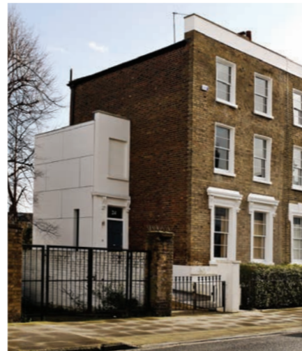
Ardleigh Road N1 - Side and rear extensions to semi-detached house in a Conservation Area
