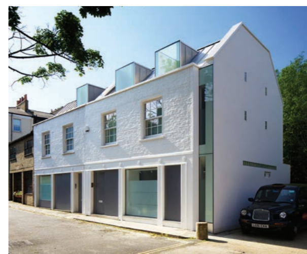
Kingstown Street, NW1 - Two neighbouring projects, both including partial rebuilds, modernisation & extensions to article 4 conservation area mews houses
