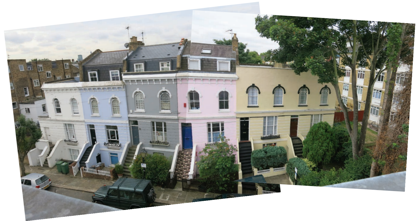
View from second floor of no.8, showing front Facade of South terrace at Baptist Gardens
