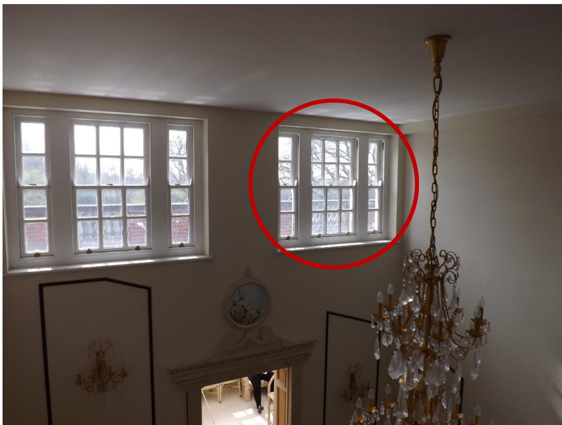
2. Internal photograph highlighting opening (opening highlighted)
