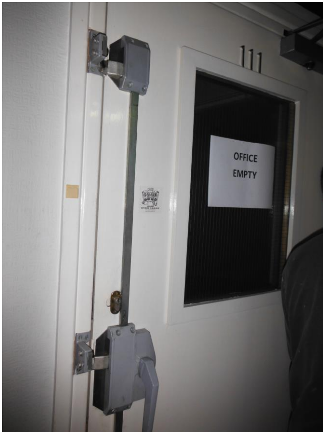
Photo 24 1 st floor room 111 (not accessed)
