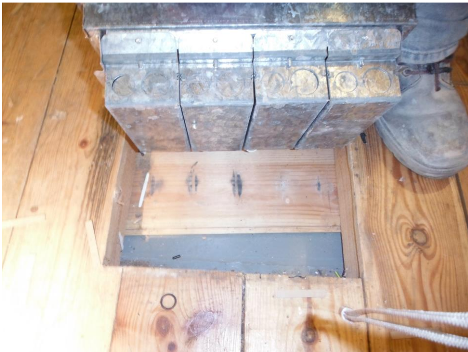
Photo 16 Ground floor Room 16 – View of concrete lower floor below wood floor.
