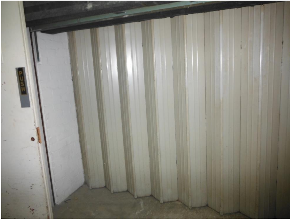
Photo 3 Lift shaft (not accessed)
