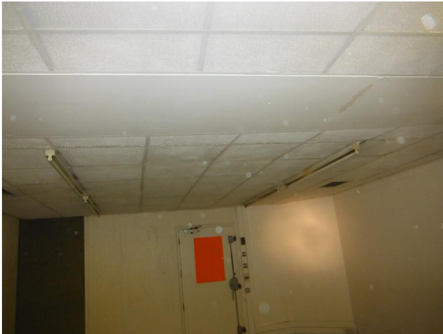
Photo 25 1 st floor room 112 – Non asbestos textured coating to suspended ceiling.
