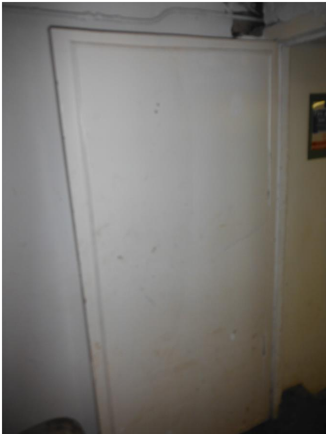
Photo 12 Basement - Asbestos cement panels lining door
