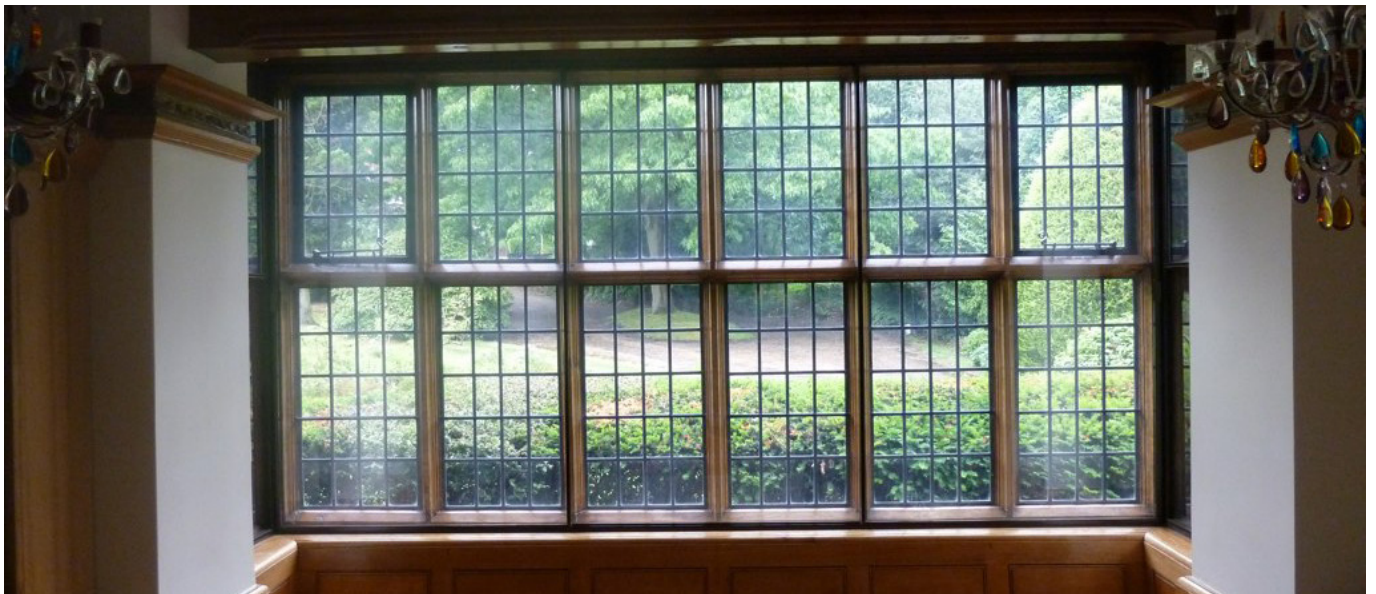
Above Examples of City Sound slimline horizontal slider system installed in front of listed windows
