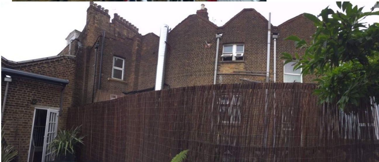
Rear elevations of properties on Kentish Town Road from back addition roof.
