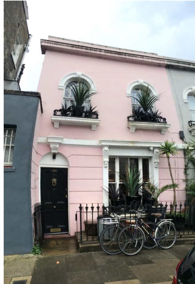
Front elevation of 1 Kelly Street.
