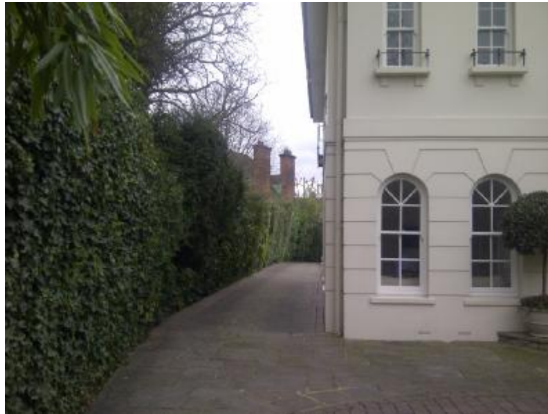
Figure 6 - The hard surfaced area to the rear of the existing dwellinghouse
