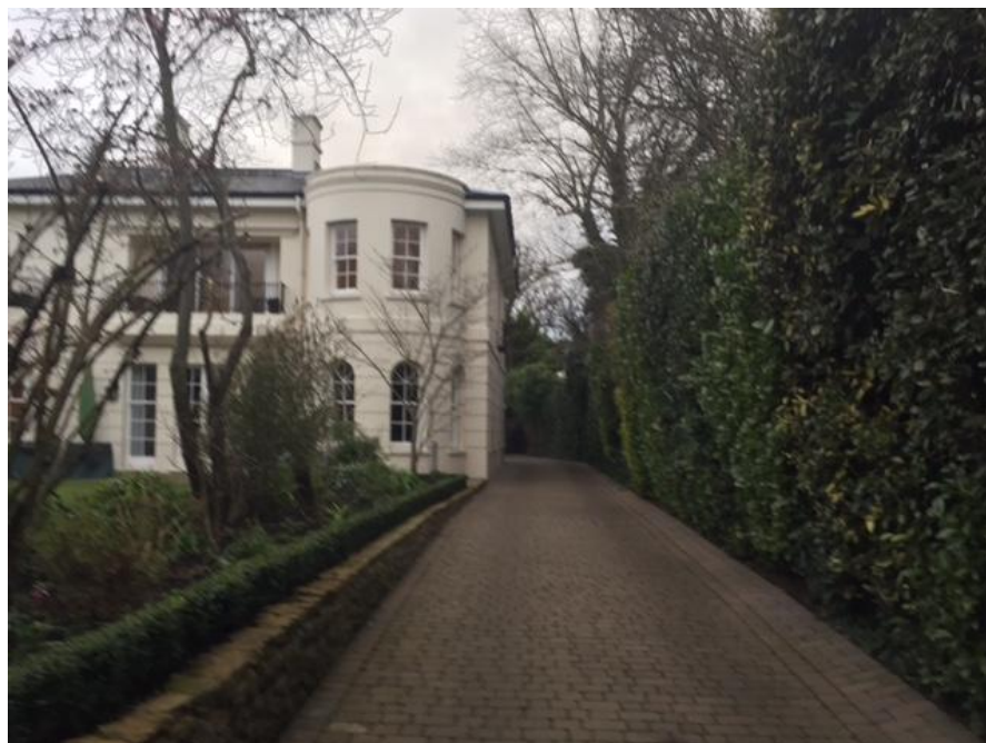
Figure 7 - The existing property is located to the rear of the plot, accessed by a long driveway
