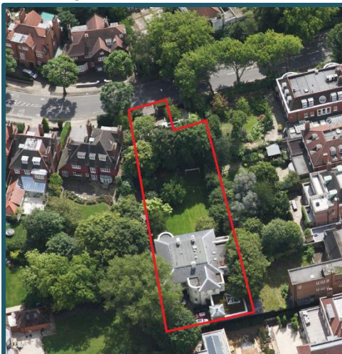
Site looking South
