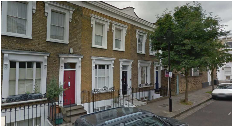
VIEW FROM THE EAST SIDE
