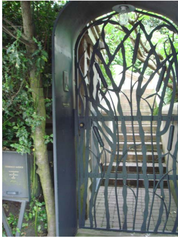
Decorative metalwork gate and mail chute, with garden shed to left concealed by hedge
