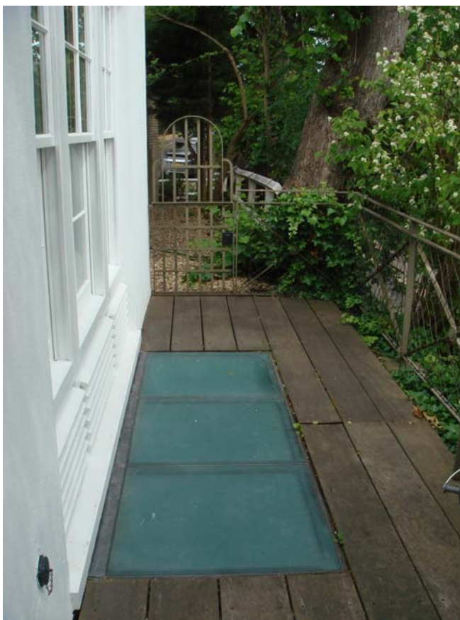
'Pavement' lights to basement in terrace adjacent to modern part of the house
