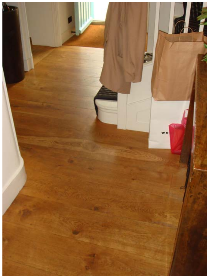
Figure 16: Oak floor installed to hall
