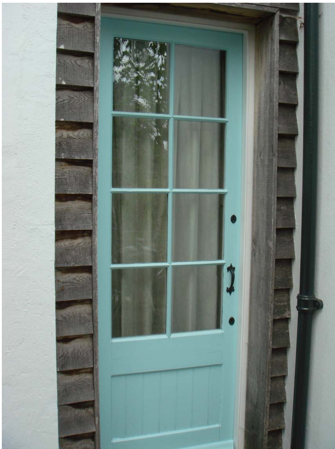
Figure 17: Timber door installed in place of approved glazed panel
