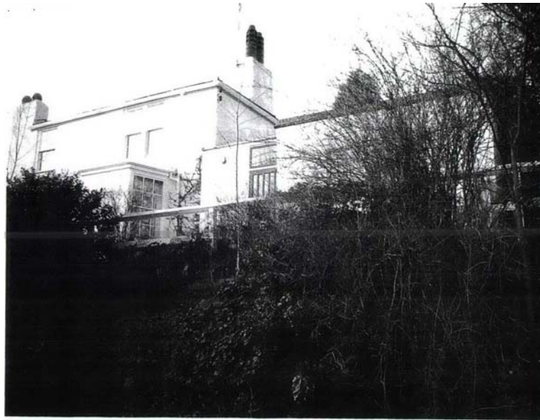
Figure 10: The rear extension as it existed in 2004 prior to works being commenced
