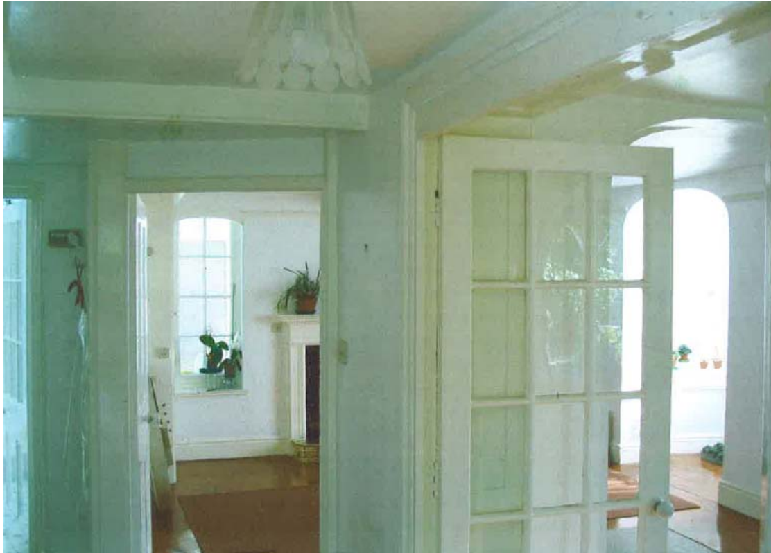
Figure 15: Double door opening (to right in image) shown prior to reduction in width to single solid door
