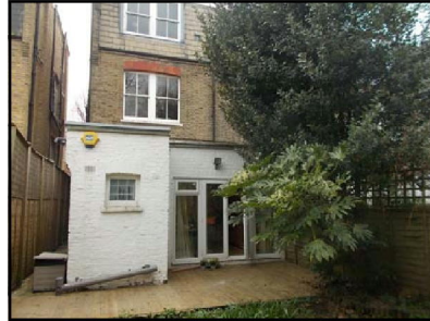
4. Rear of the property showing S1 and T8.
