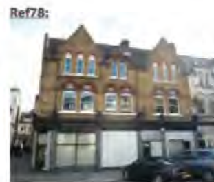
Ref78: Mid to late 19th century 3 storey building with retail at the g/f. The g/f has substantial alterations to the main shop fronts but the console brackets remain in situ and carry along the length of the property. At second floor level window are set back within a stilted brick semicircular arch with mosaiced spandrel.
