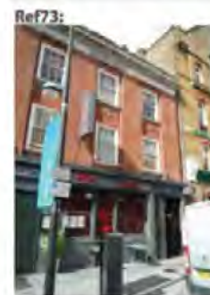
Ref73: Former pub and now restaurant. This pub dates back from the early 19th C. The building has the dates 1837 to 1901 on the parapet. The windows are set back within framed columns
