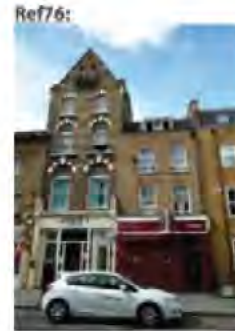
Ref76: Mid to late 19th century 4 storey building with 5th floor built into the gable face of the pitched roof and retail at ground floor. The front elevation has an eclectic range of detailing adding to its significance as a unique addition on this street.
