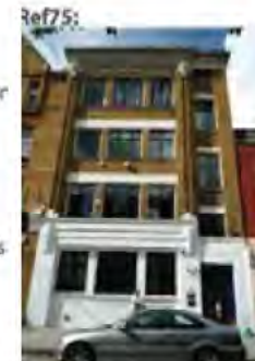
Ref75: Erected between 1935 and 1953 and was used as part of 39 to 41 (industrial). The building seems to follow an art-deco style in its detailing whilst keeping the verticality and floor levels of the 39 and 41.
