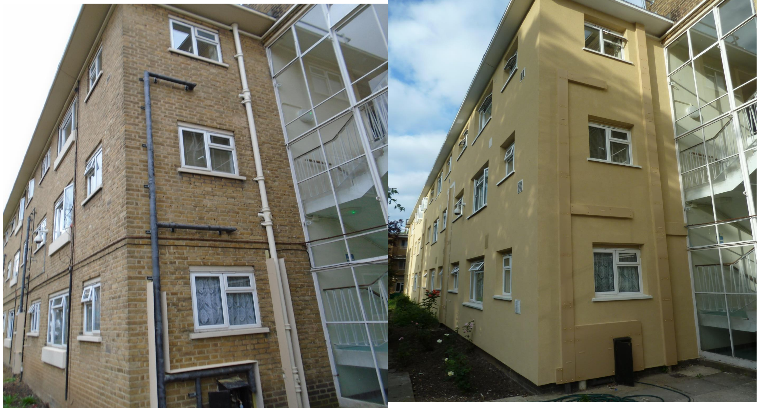
1-48 Greenwood, Oseney Crescent Before and after pictures showing boxing of downpipes.
