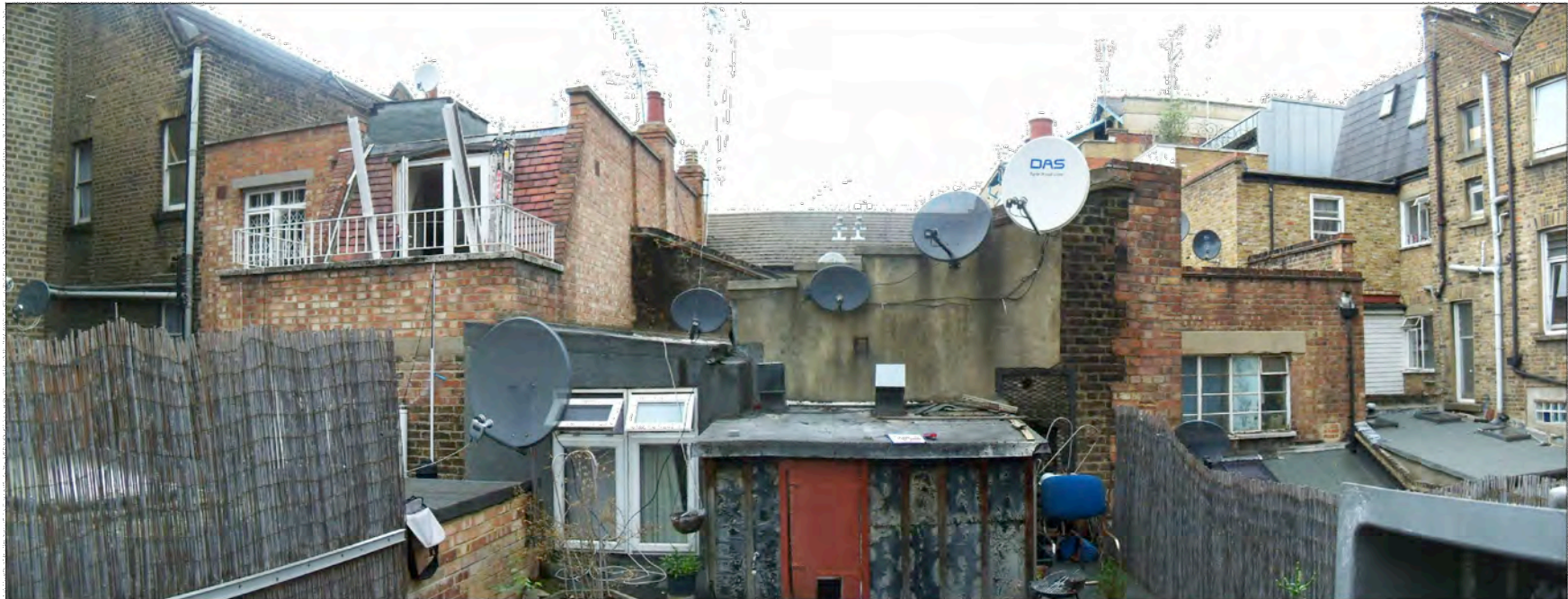
Existing Rear Photos
