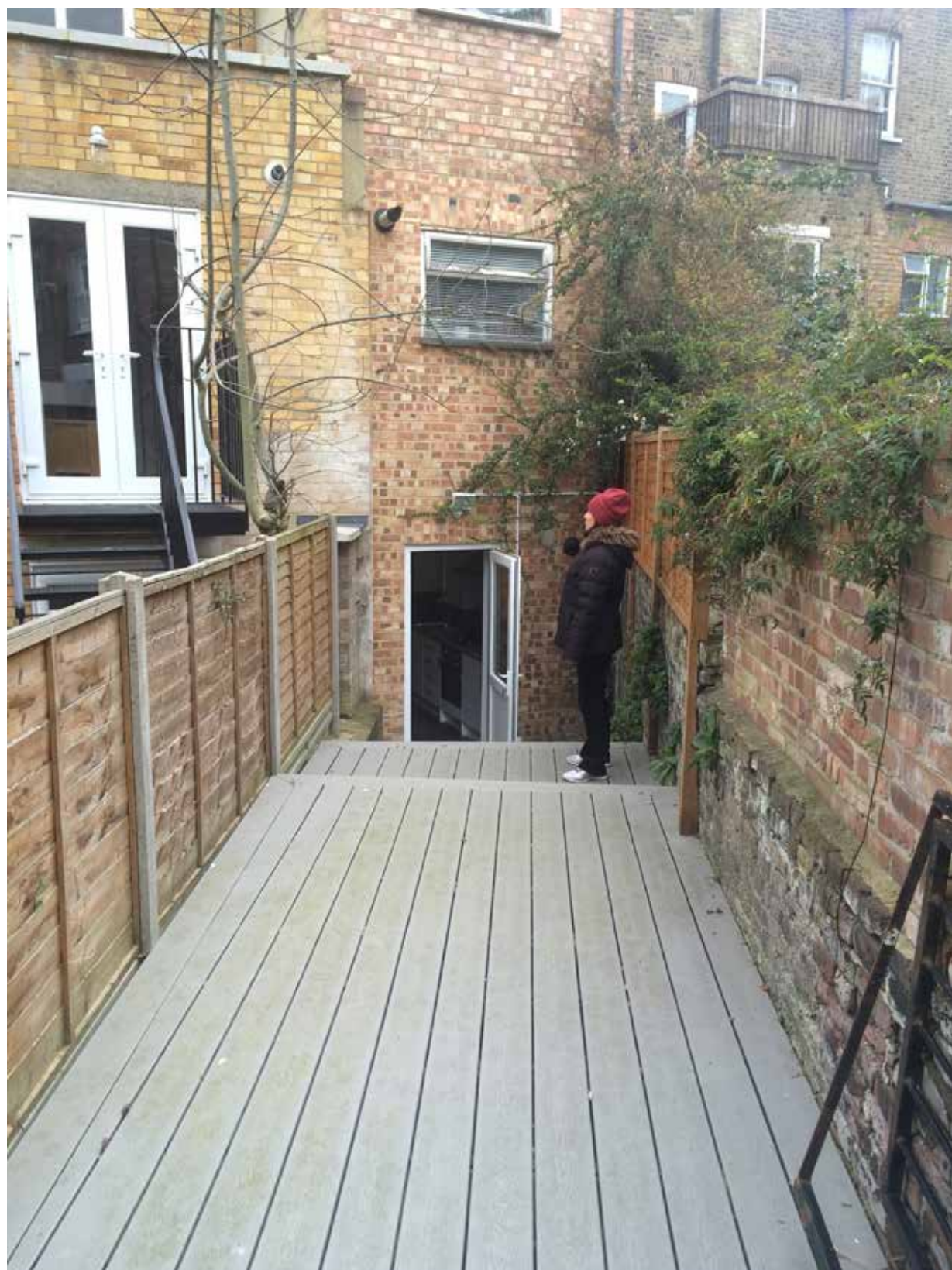
Existing Rear Patio and 90 Torriano Avenue Rear Facade
