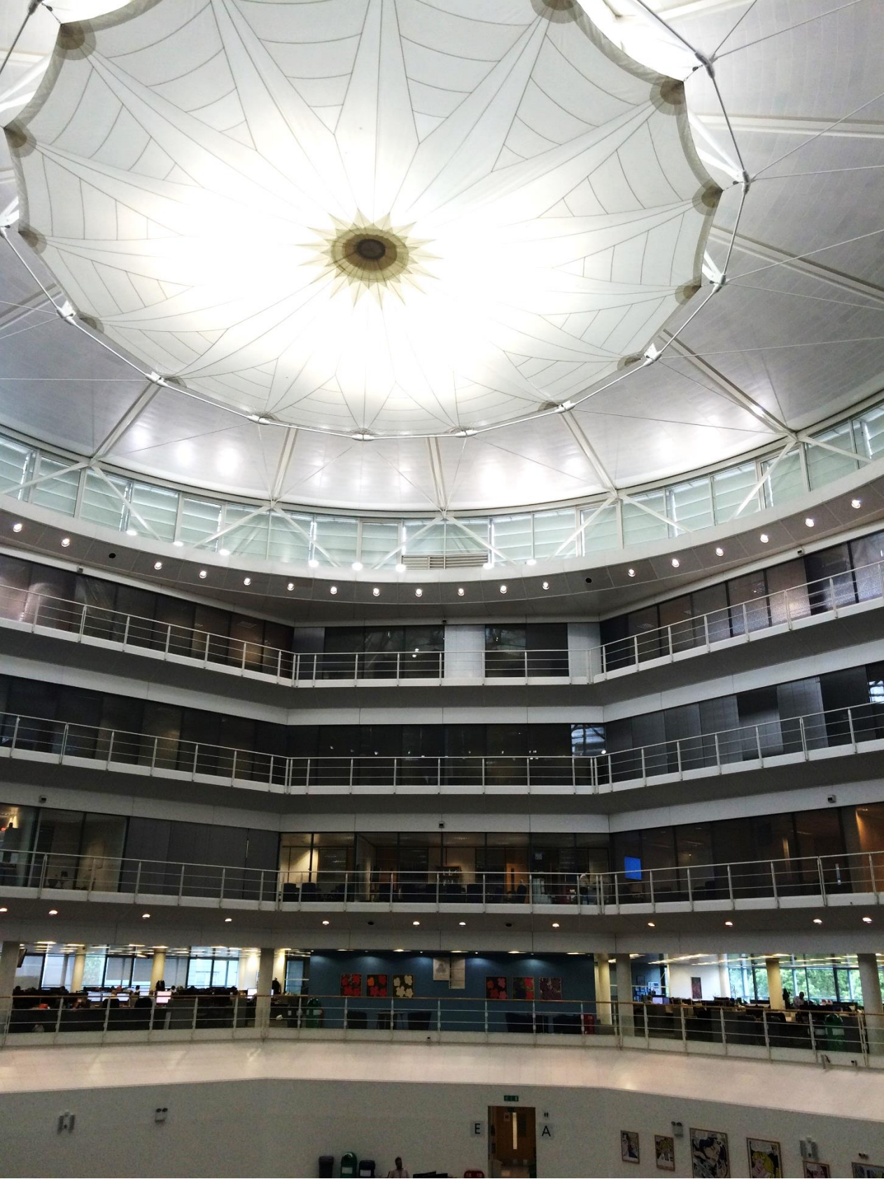
view of existing atrium including suspended internal roof structure taken from 2 nd floor on 4/9/2015
