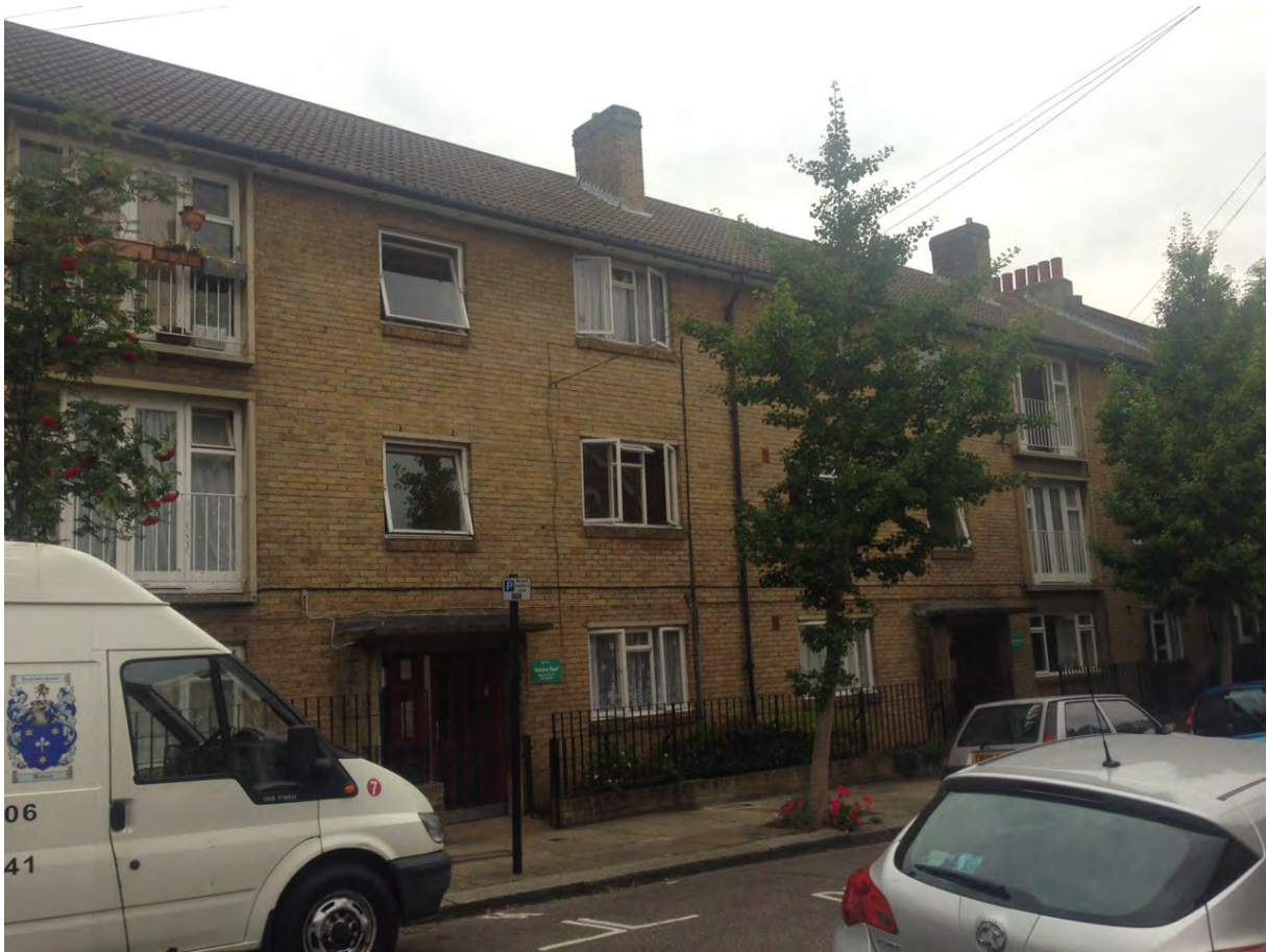
Modern Infill Block - 25-35 Twisden Road
