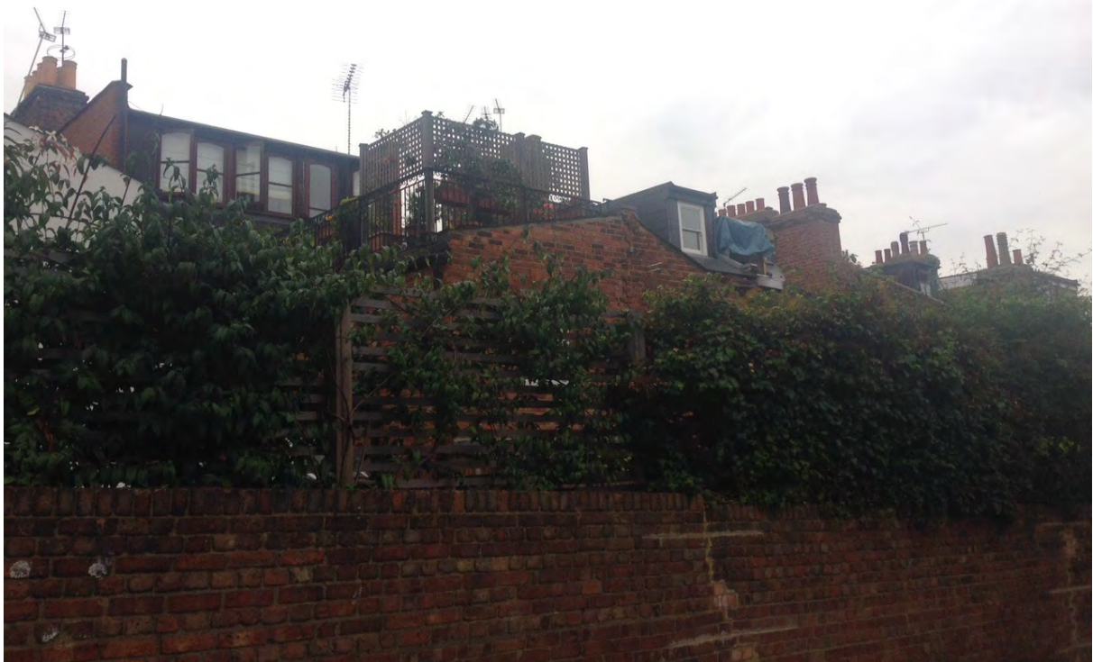
Rear of Nos 60-74 Twisden Road showing new Dormer extension at No.66
