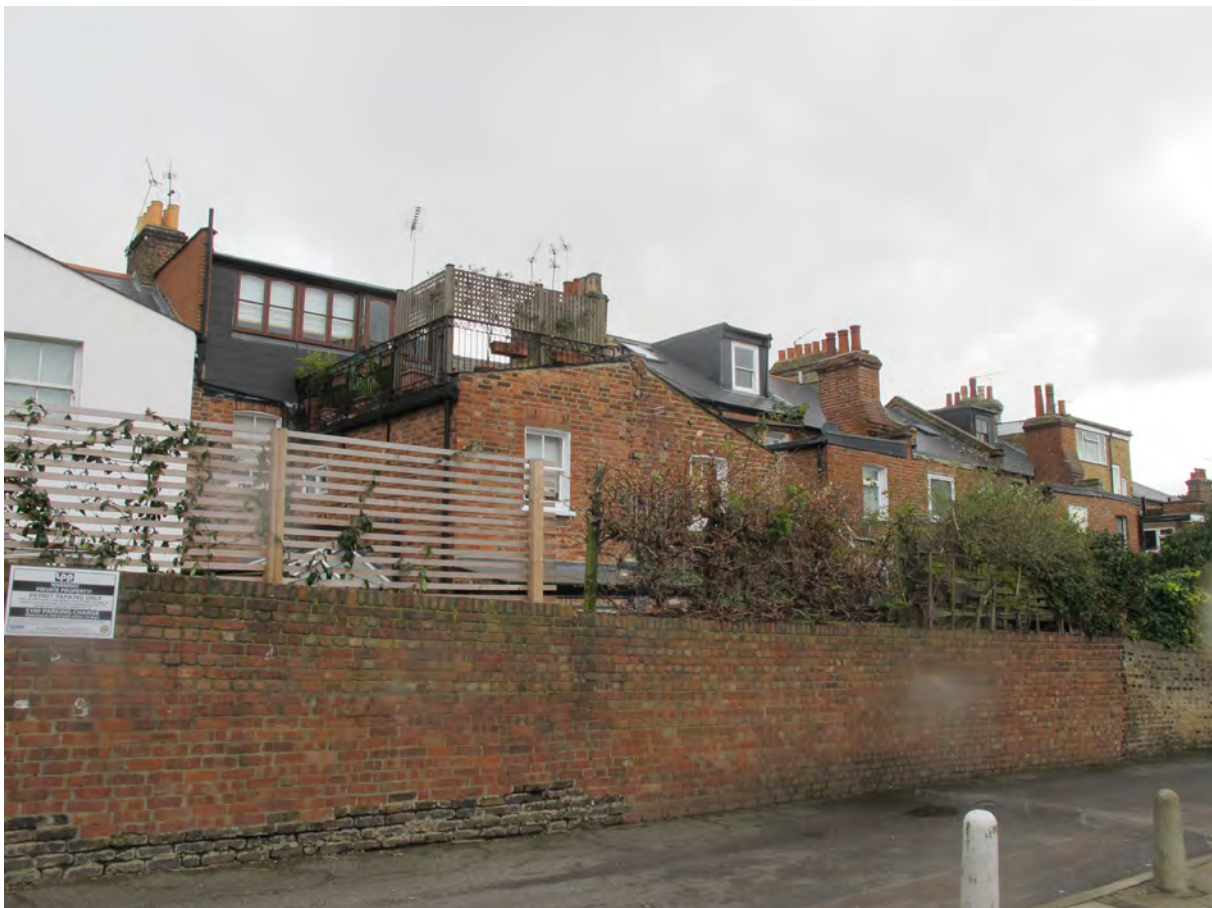
Rear of Nos 60-74 Twisden Road (prior to construction of new Dormer at No.66)
