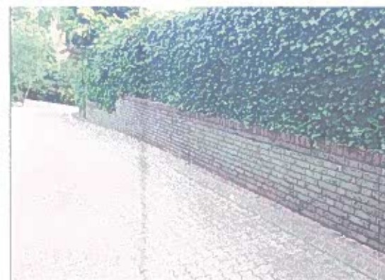
PHOTO 8 Existing fence brick wall
