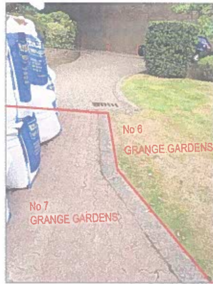
PHOTO 2 Existing entrance front patio
