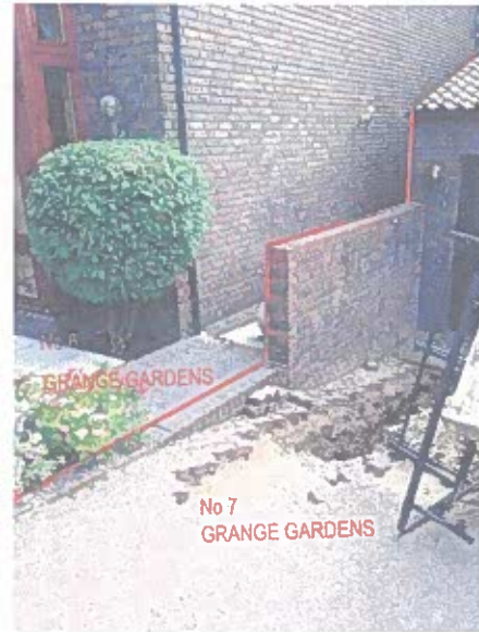
PHOTO 1 Existing fence brick wall
