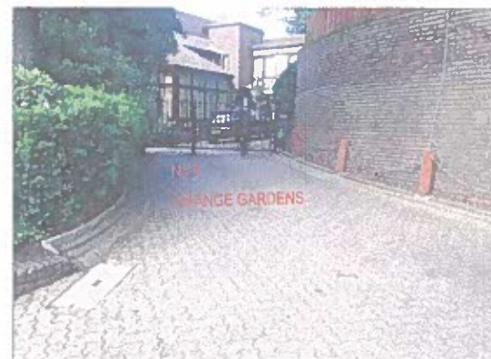
PHOTO 7 Existing fence brick wall
