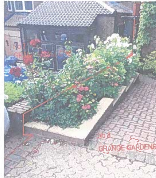
PHOTO 3 Existing fence brick wall
