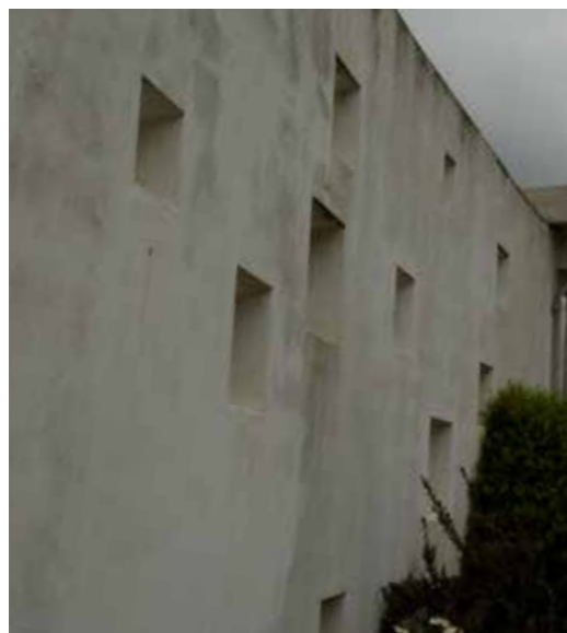
Fig. 10-12 existing view of ancillary buildings
