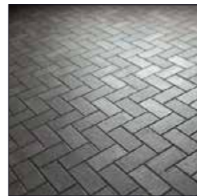
"staffordshire blue" brick slips laid in herringbone pattern on existing substrate
