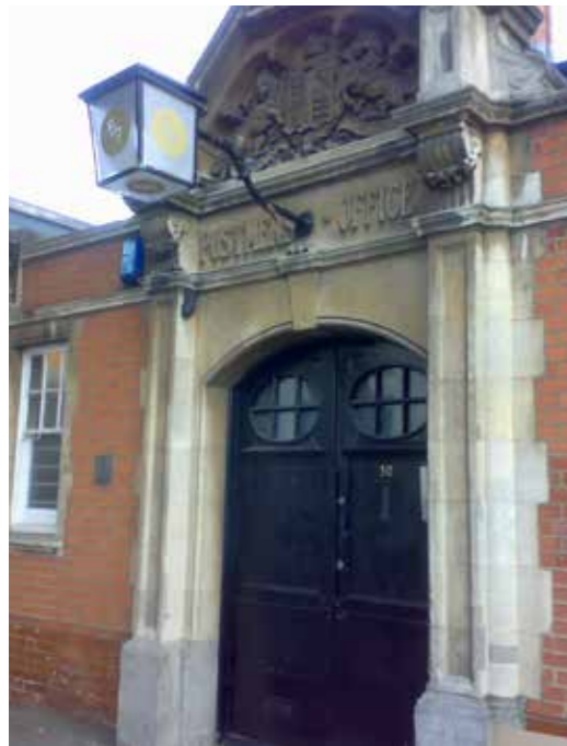
Fig. 4 existing frontage of brick and portland stone
