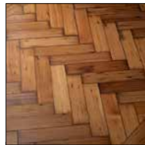
existing pine parquet floor in herringbone pattern to be refinished where shown, all areas lifted to be carefully set aside for reuse within the building.
