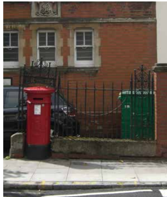
Fig. 5 existing bespoke railings to Leighton Rd
