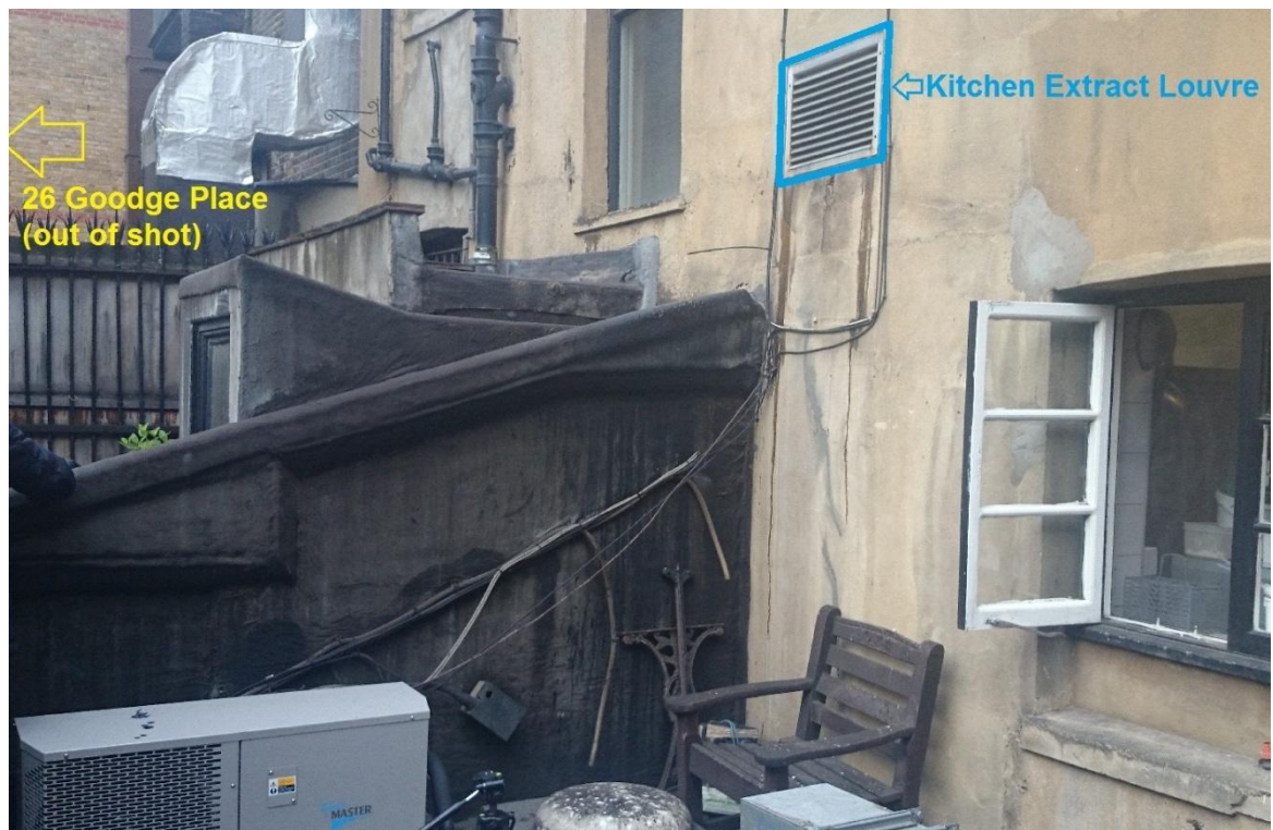
Figure 5.1: Photograph showing the location of The One Tun kitchen extract louvre
