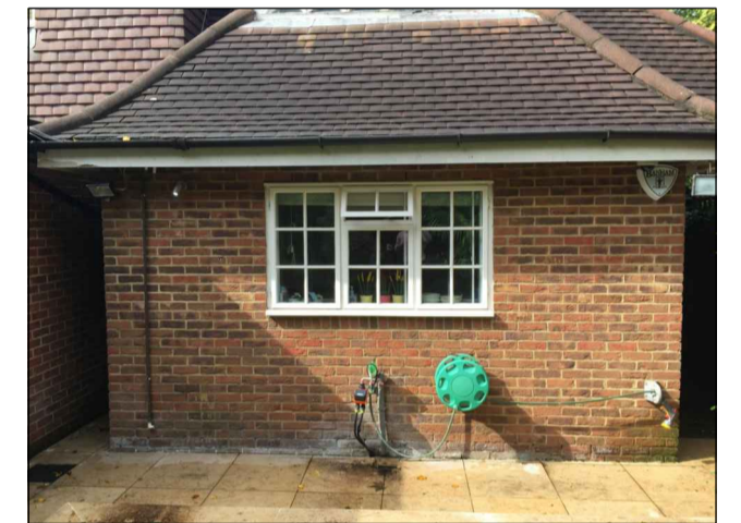
Photo Showing Existing Rear Window To Be Replaced
